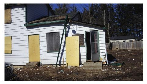
Figure 2 – Detached gutter
