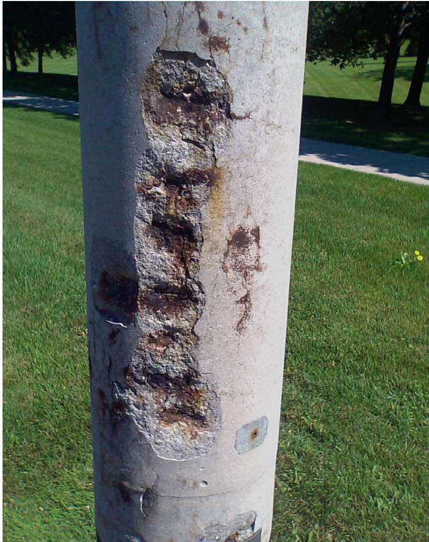
CONCRETE SPALLING, RUSTING, EXPOSED REINFORCING BARS
