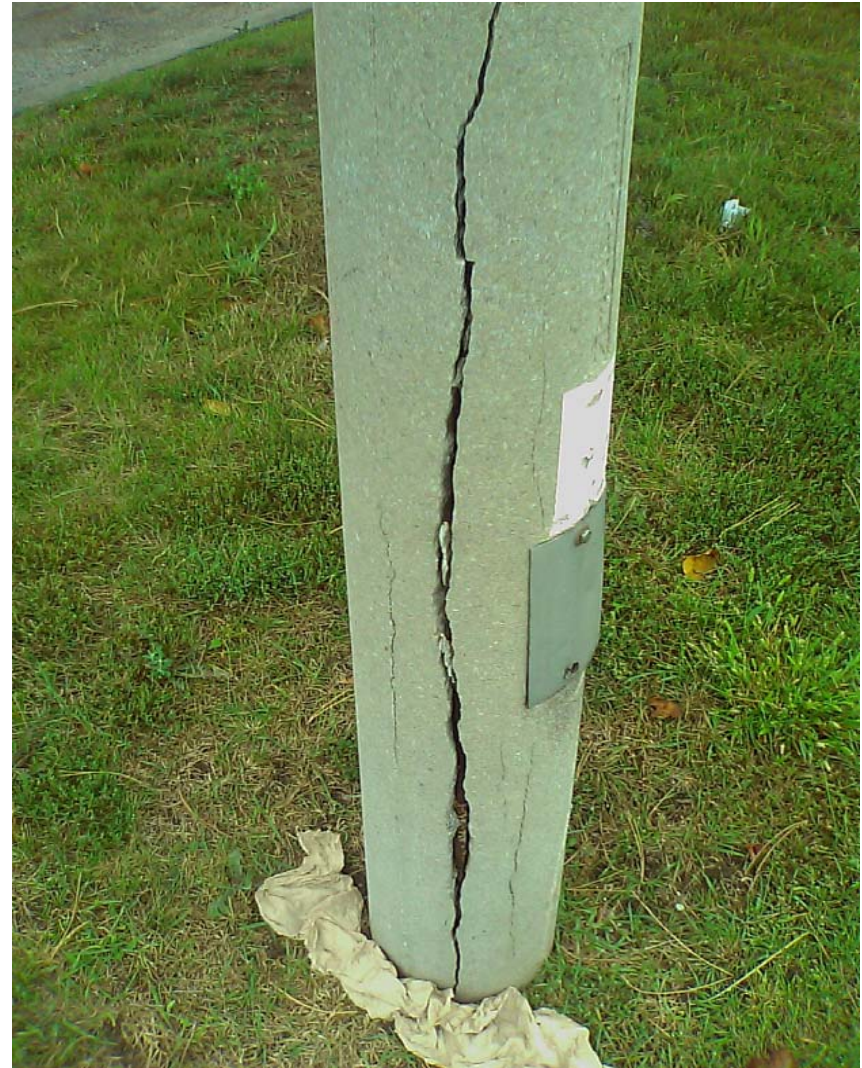
CONCRETE CRACKING
