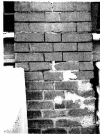
Progressive deterioration: Rainwater splashing on the porch and steps eroded the mortar. That let increasing amounts of water into the bricks and mortar below, and they are spalling and washing away, letting in even more moisture.
