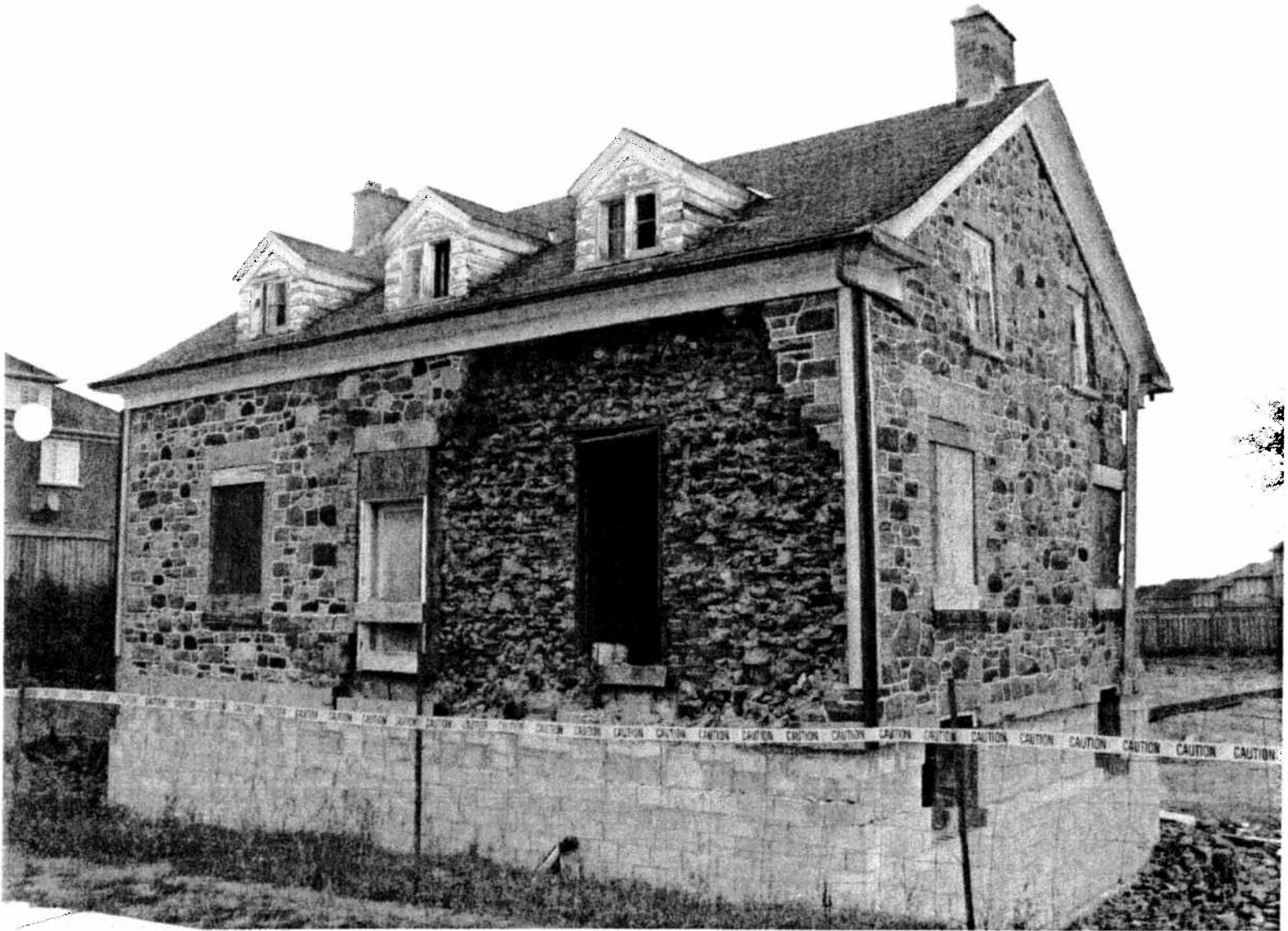
Robb House, damage to front wall following relocation. (2007 photo)
