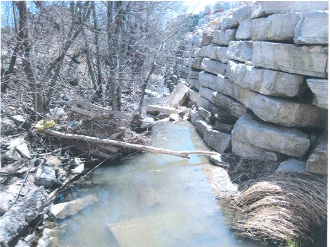
Figure 22(b) - Reach of Pomona Mills Creek Downstream of 1800 mm Diameter Culvert (Looking Downstream)
