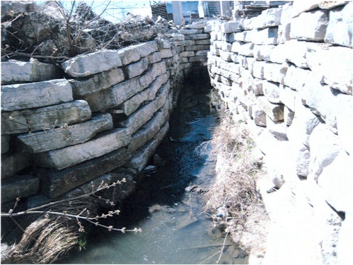
Figure 22(a) - Pomona Mills Creek at Outlet of 1800 mm Diameter Culvert (Looking Upstream)
