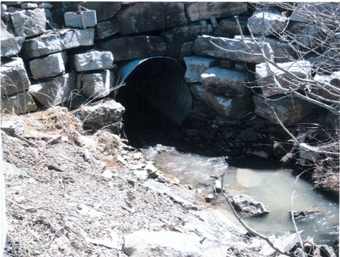
Figure 21 - Entrance of 1800 mm Diameter Culvert
