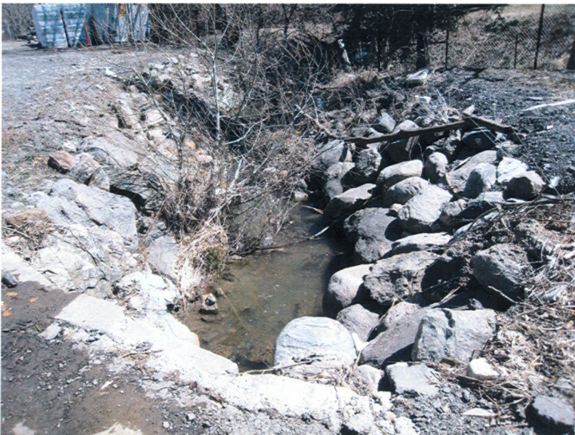
Figure 24 - Outlet of 900 mm Diameter Culvert
