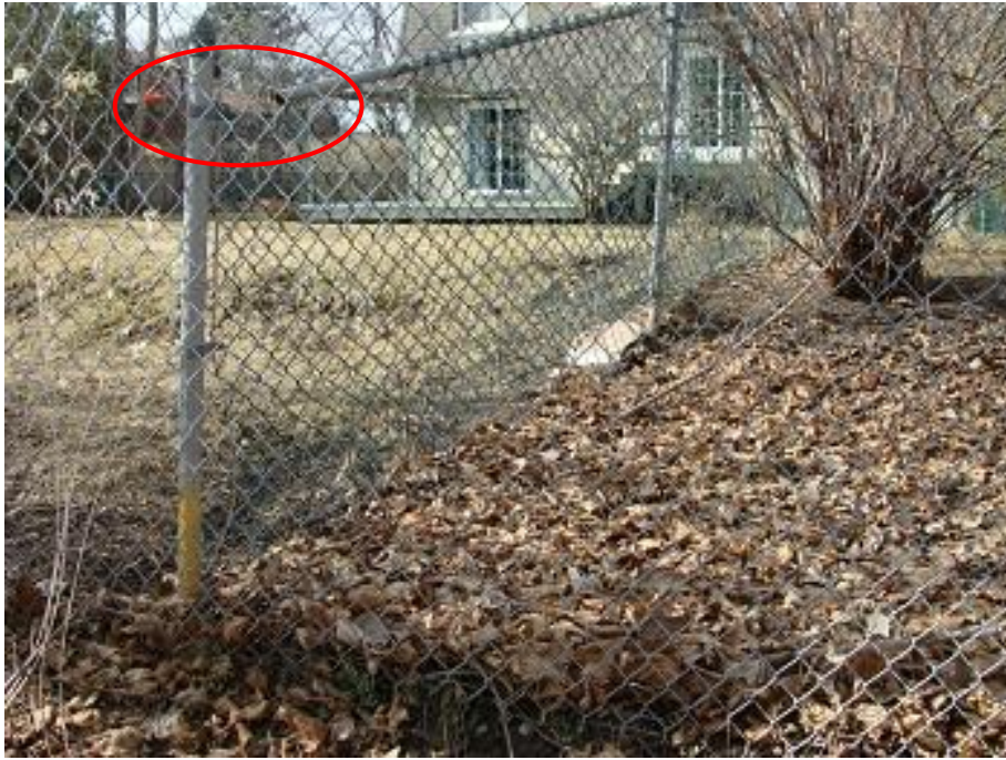
Landfill settlement #2 (fence pole shifted)
