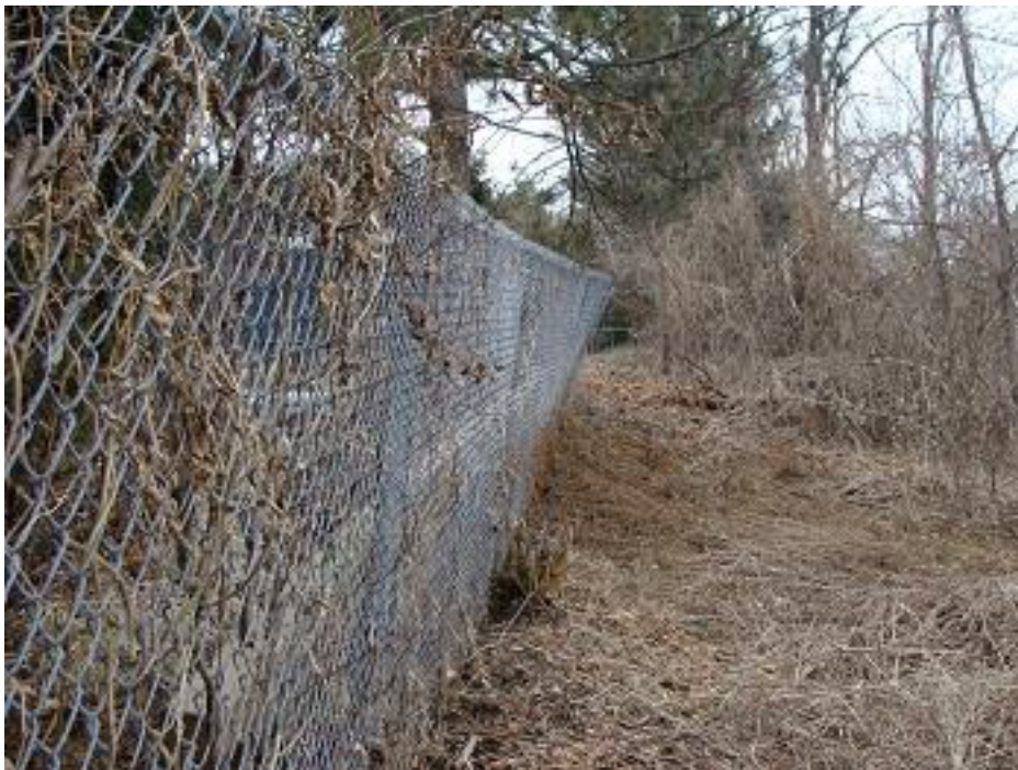
Landfill Settlement #3 (fence pole shifted)
