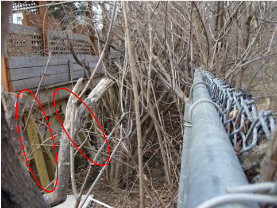
Landfill Settlement #4 (gazabo foundation shifted, extra supports required )
