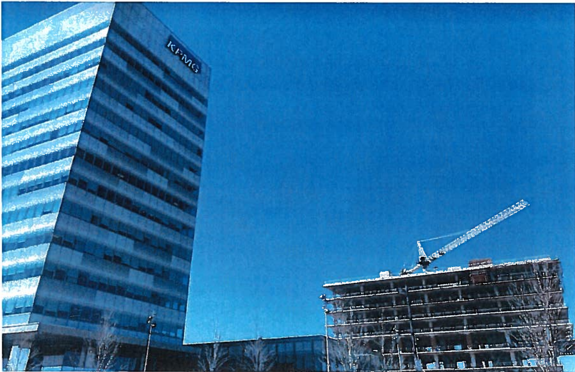
Figure 10 Construction activity in the Vaughan Metropolitan Centre, April 2018
