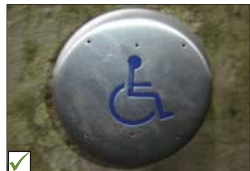
Figure 40b: Touch Activation Device - Elevation View
