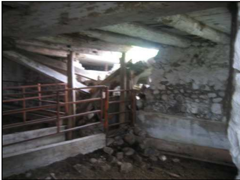
Photograph 31: Collapsed foundation wall
