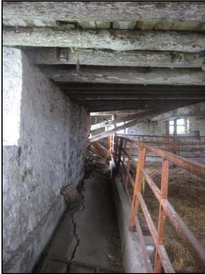
Photograph 36: Damaged floor slab
