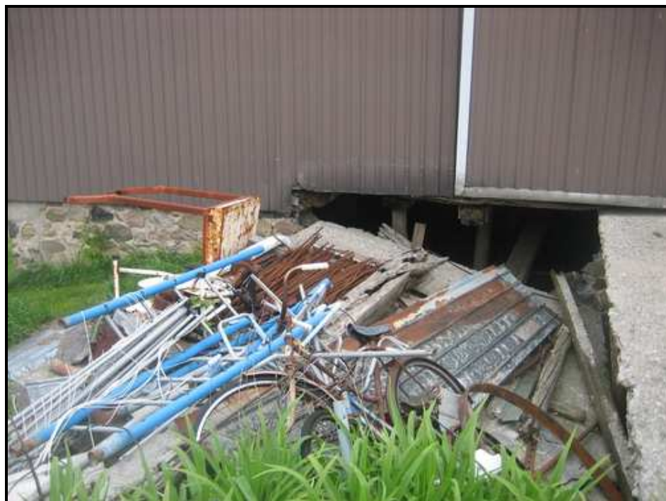
Photograph 30: Collapsed slab
