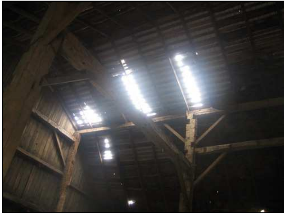
Photograph 34: Roof panels missing
