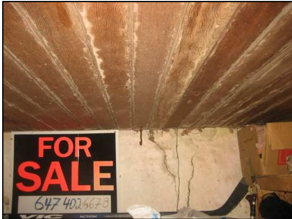
Photograph 29: Crack in interior parging
