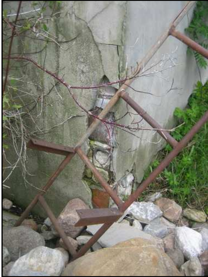
Photograph 37: Damaged clay tile foundation
