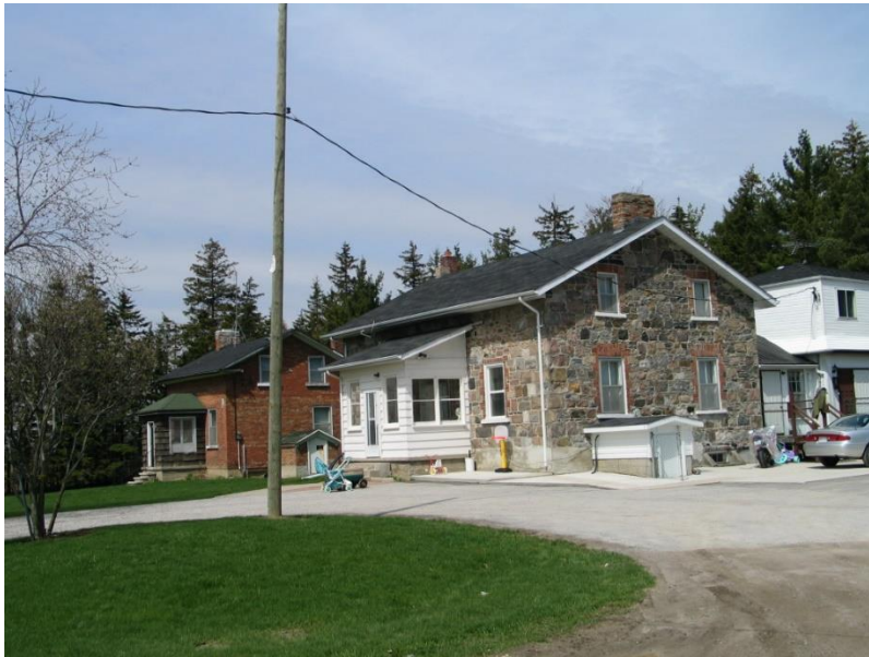
10535 and 10537 McCowan Road, showing the relationship between the two dwellings. Note the exterior cellar entrances.
