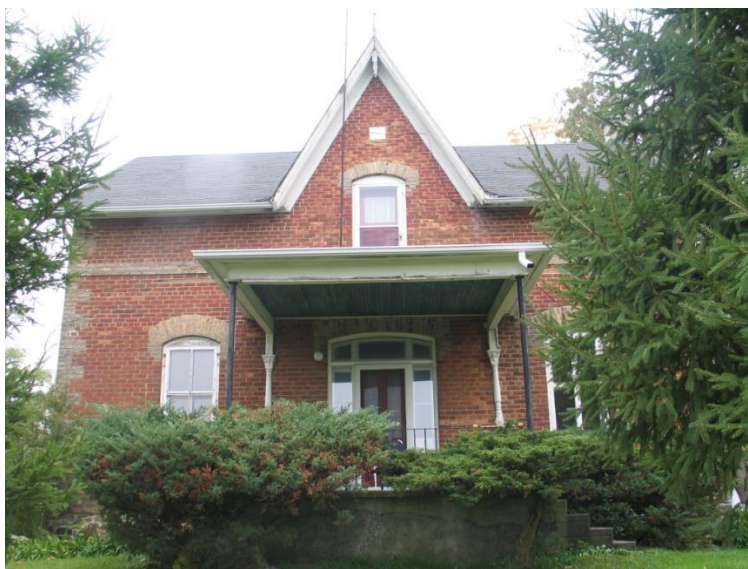
Detail of East (Front) 10224 Highway 48
