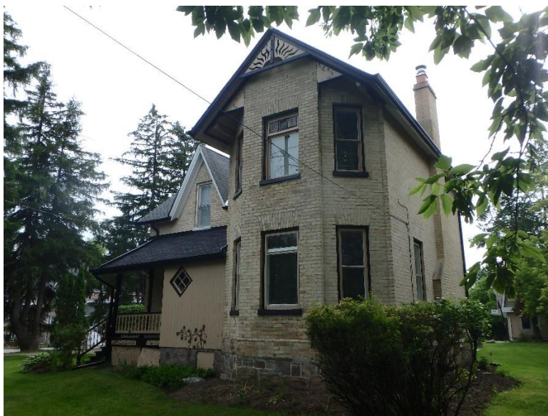
East and North Sides of 7530 Ninth Line.
