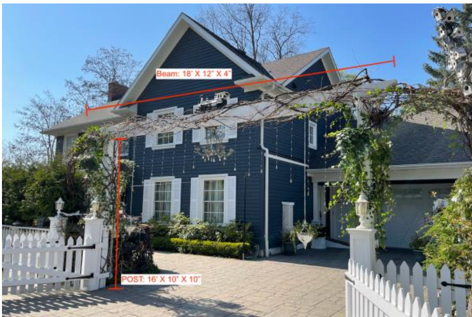
Primary (south) elevation of 146 John Street showing the recently constructed driveway arch (Source: Applicant c.2024)
