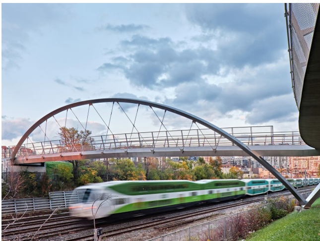
Figure 138. Bridges can provide a great way for pedestrians and micro-mobility users to cross major obstacles.
