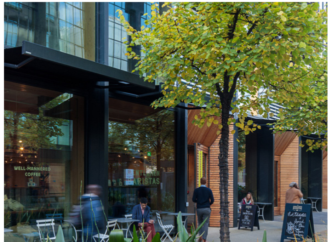
Figure 151. Mid-rise buildings can help transition with stepbacks to and mitigate shadowing, adverse winds and overlook.
