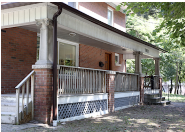
Figure 102. Front Porch of 7951 Yonge Street.
