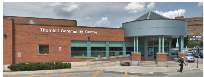
Figure 62. Thornhill Community Centre.
