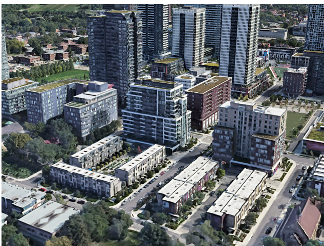
Figure 148. Taller ground floor heights can offer the opportunity to retail and employment use to relate better with the public realm.
