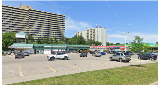
Figure 54. Low-Rise Retail Plaza and Food Basics at Yonge Street and Royal Orchard Boulevard with surface parking.
