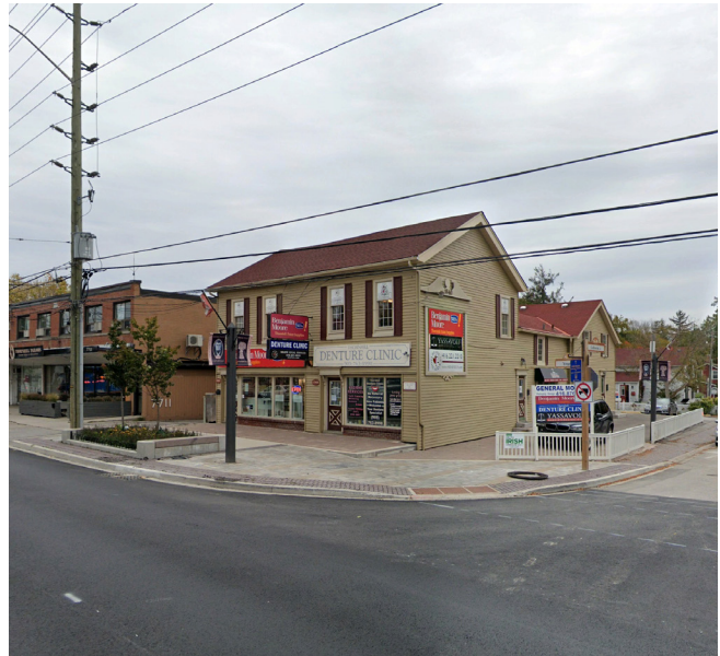
Figure 100. Low-rise heritage property containing retail uses along Yonge Street.
