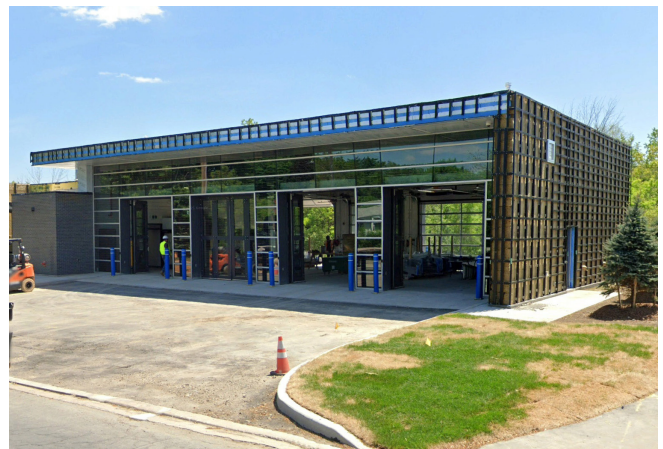
Figure 71. York Region Paramedic Response Station - 29, located along Glen Cameron Road at the northeast corner of the employment lands.
