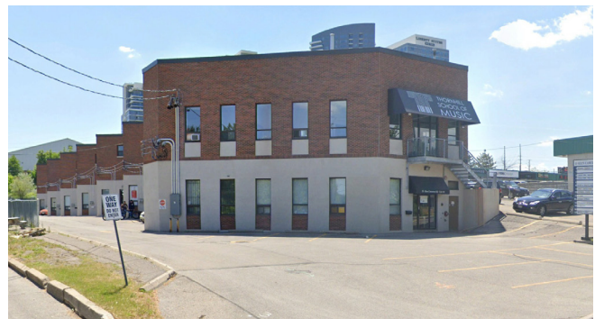
Figure 50. Light industrial and local service uses adjacent to the rail corridor.
