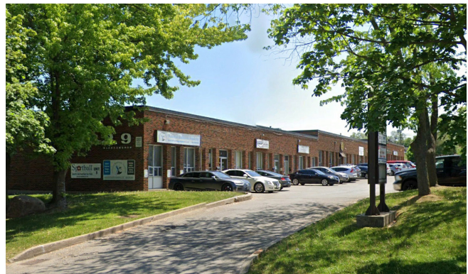
Figure 41. Light industrial and local service uses adjacent to the rail corridor.
