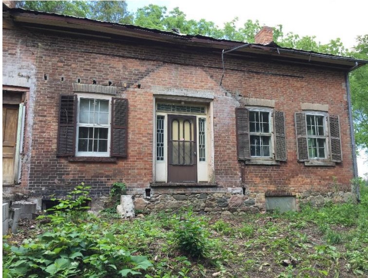
Front view taken in 2021 with doddy house removed. Note the door on the left, originally a window.
