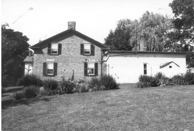
East side view from 1981 showing rear addition.
