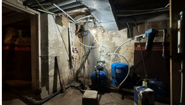
Retrofit HVAC Fixtures & Concrete Parging
