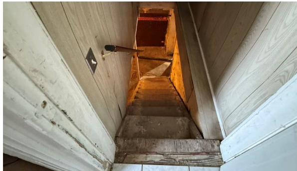
Staircase to Basement
