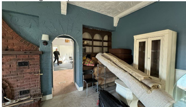
Living Area (Addition on South Side)
