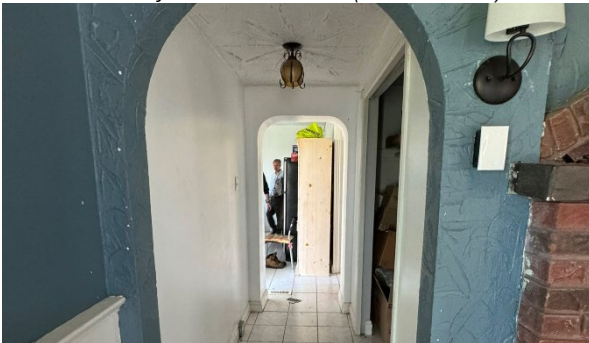
Hallway from Addition (South Side)
