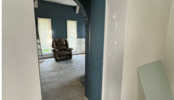
Wall Thickness Between Original & Addition
