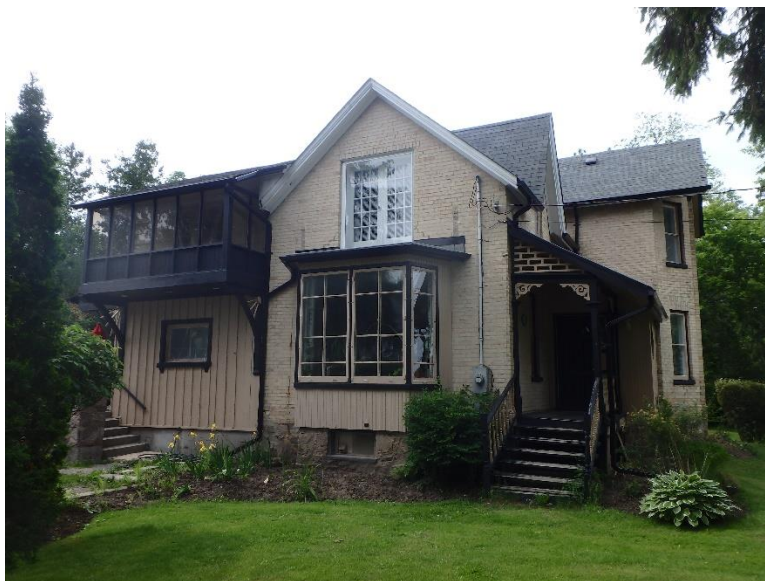
South side view of 7530 Ninth Line showing veranda detailing, south bay window and rear addition.
