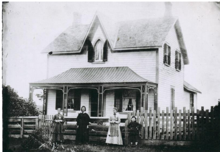
Archival photograph of the Frisby House showing clapboard siding and bellcast-roofed veranda. Markham Museum Collection.
