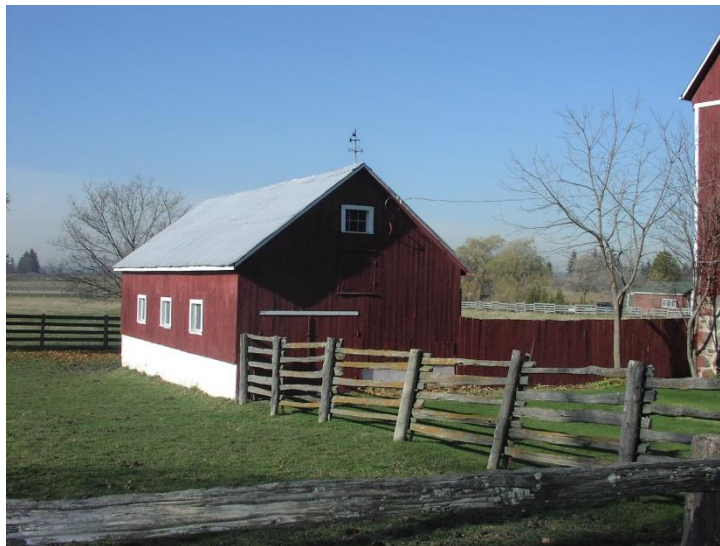
Shed at 3812 Nineteenth Avenue.
