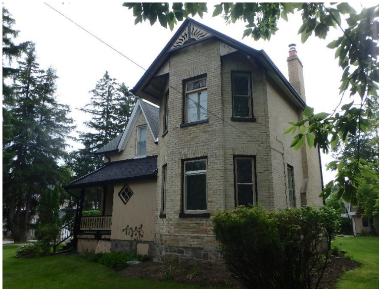
East and North Sides of 7530 Ninth Line.
