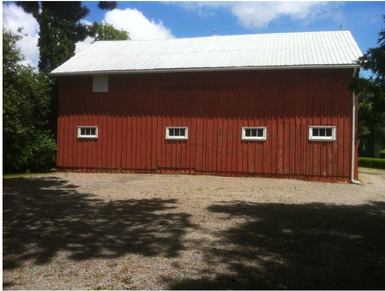
Barn at 3693 Elgin Mills Road East, prior to alterations in late 2010s. This building may have served as John Doner's carpentry shop.
