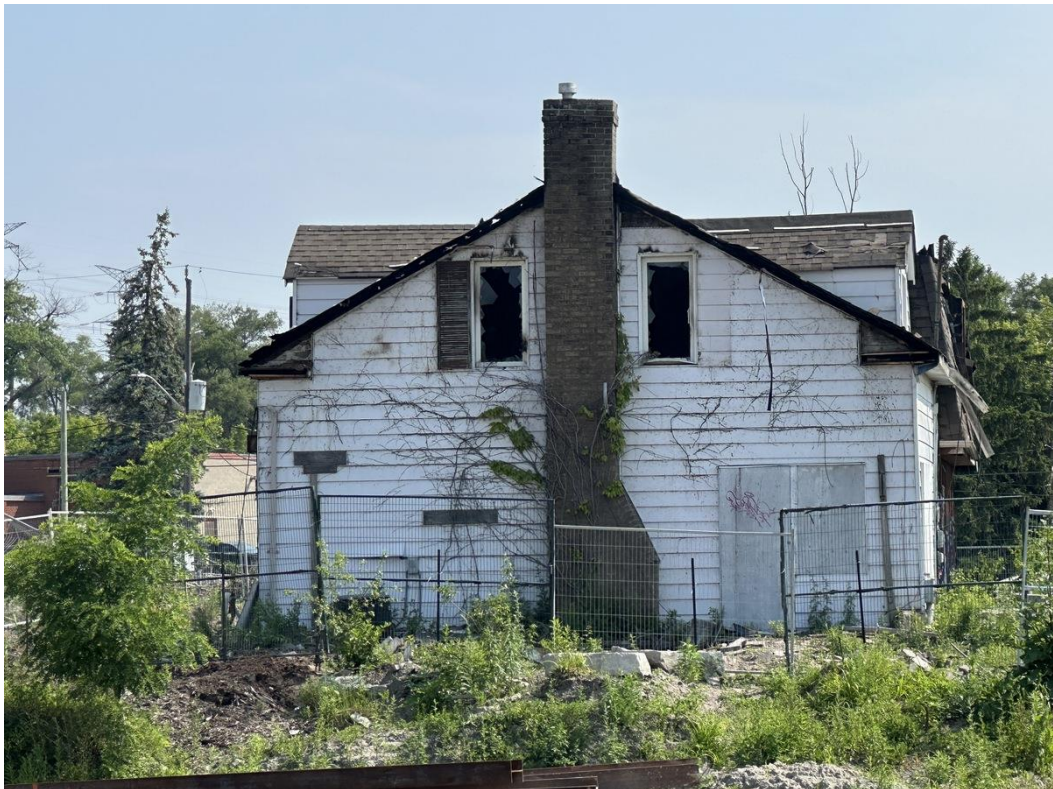
Photo 2 – View of West Elevation
