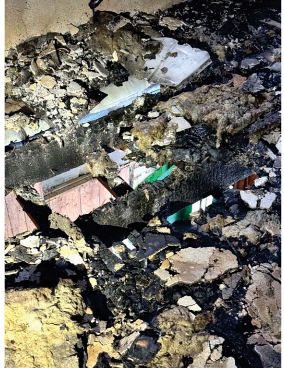
GROUND FL JOISTS AND SHEATHING
