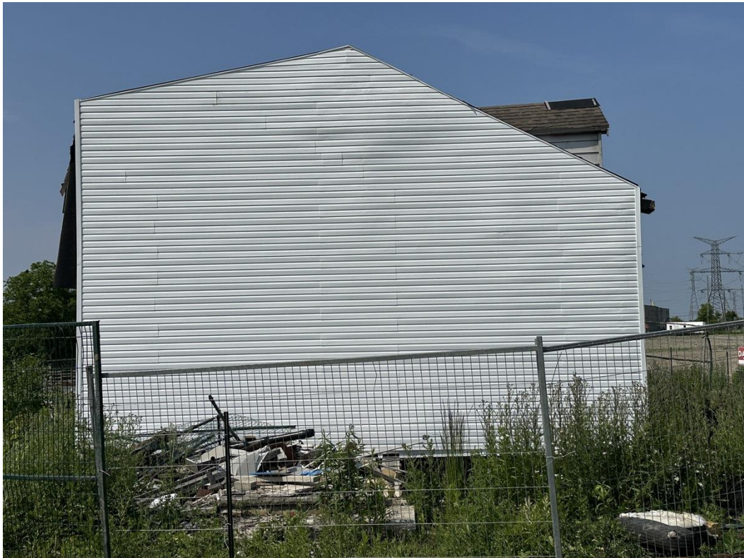
Photo 4 – View of West Elevation
