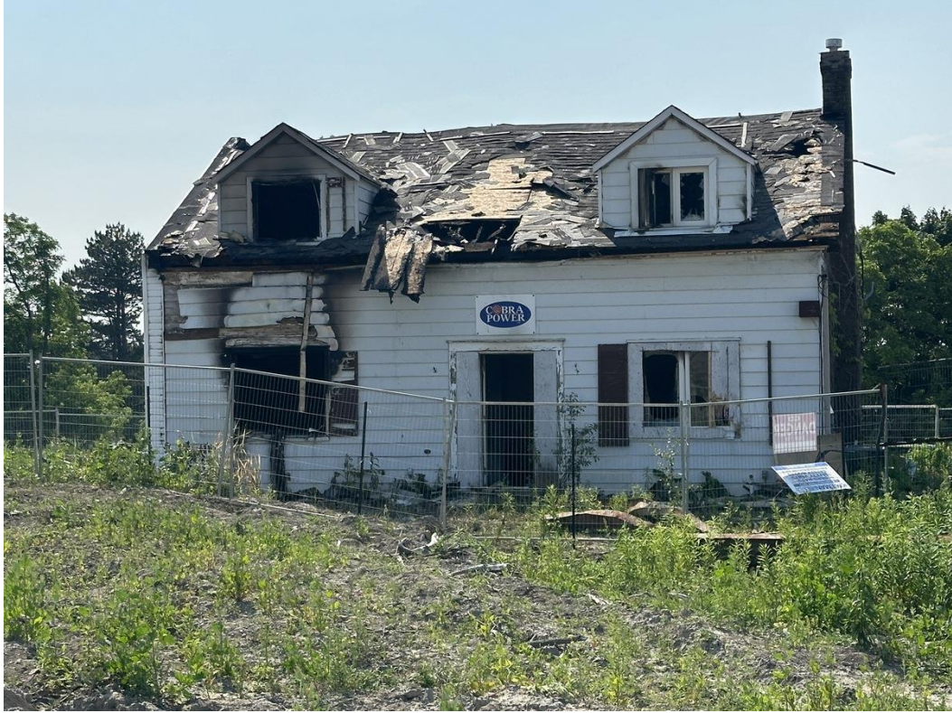
Photo 3 – View of North Elevation
