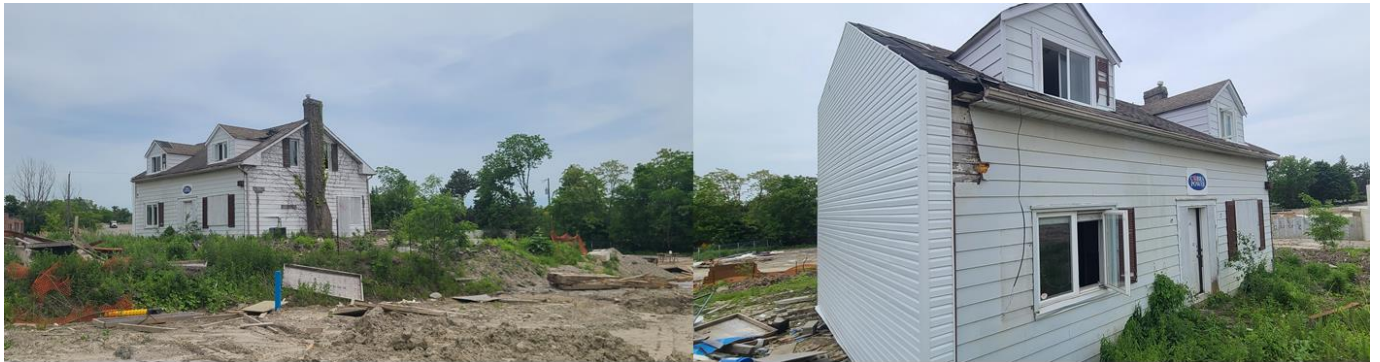
After the removal of the newer addition
