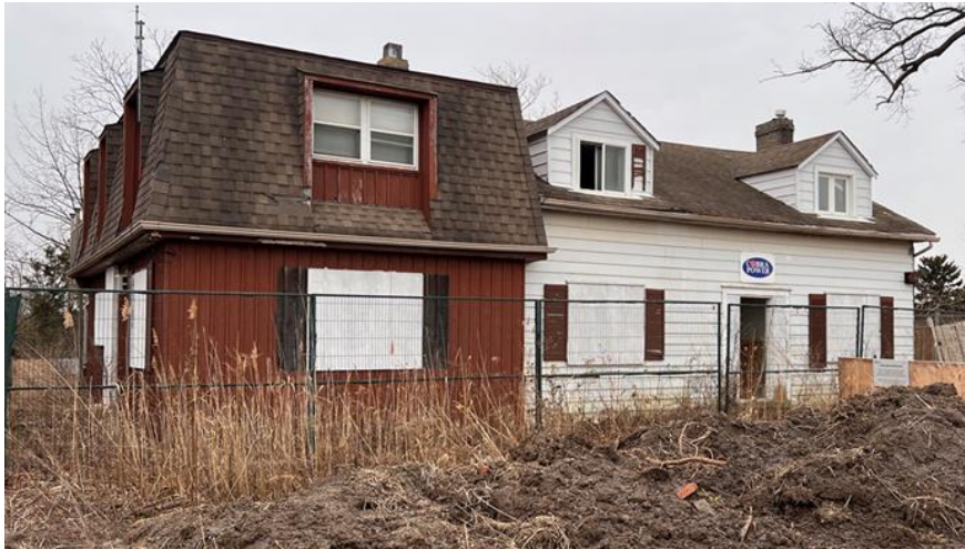
Prior to the removal of the newer addition
