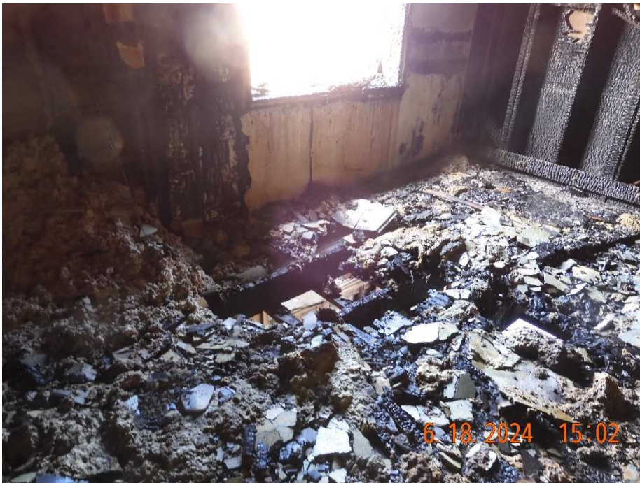
Ground floor level @ north east corner of building
