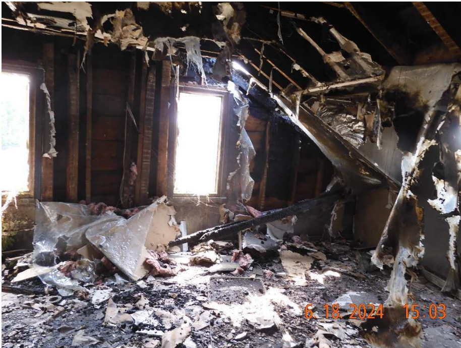
Roof level @north west corner of building (from 2 nd floor level)
