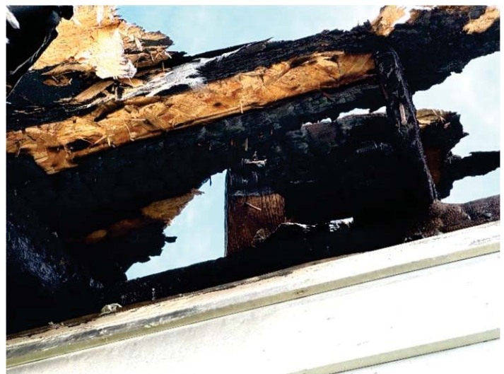
RAFTER TAIL AND SOFFIT FRAMING
