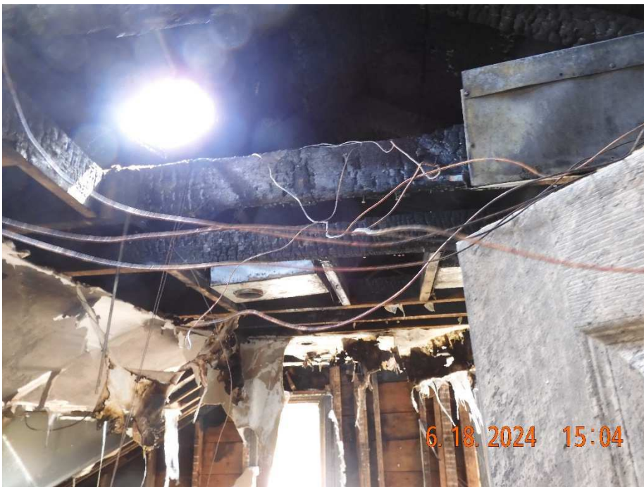
Roof rafter & collar tie (from 2 nd floor level)
