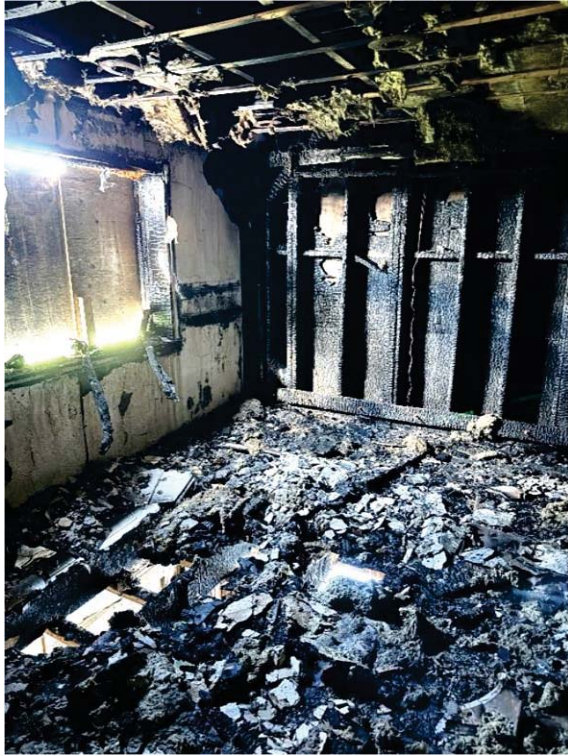
GROUND FL LOOKING NORTH EAST
