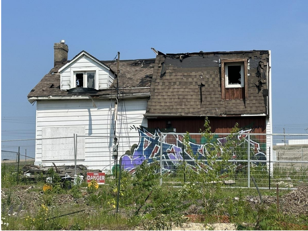
Photo 1 – View of South Elevation
