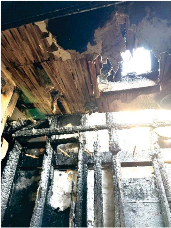
SECOND FL AND CEILING FRAMING
