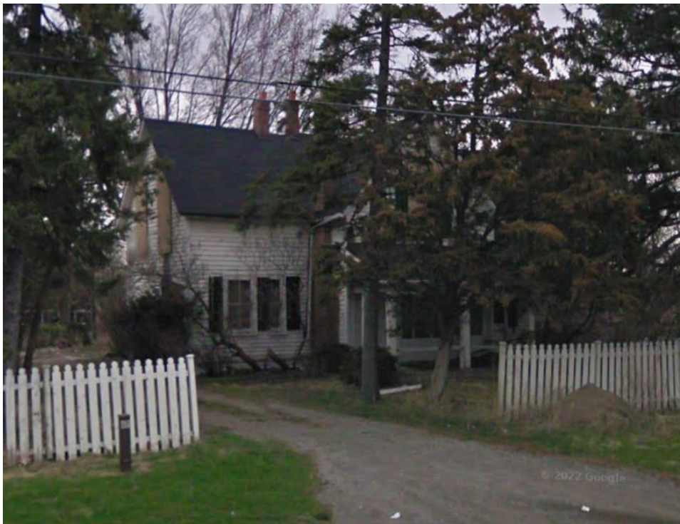
2977 Sixteenth Avenue outlined in blue [above] and an image of the dwelling's primary (north) elevation [below] (Source: City of Markham, Google)
