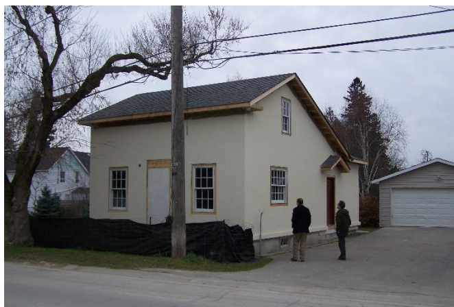
10754 Victoria Square Blvd as renovated between 2006 and 2011. Source: City of Markham
