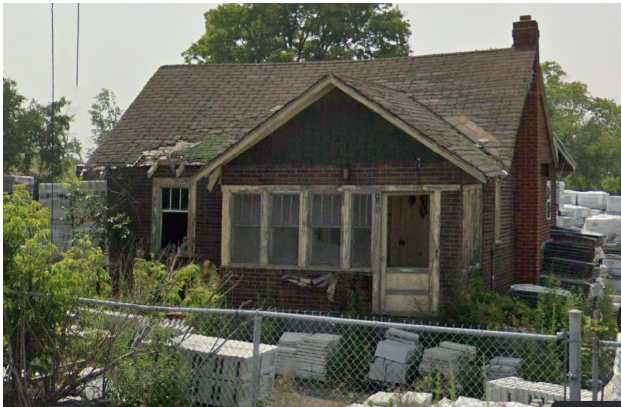
Primary (north) elevation of 139 Langstaff Road East (Source: Google, June 2023)
