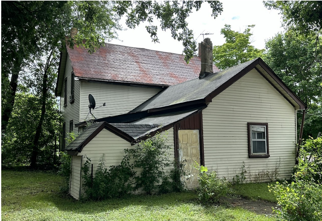
Figure 7 - Rear (west) elevation of 11534 McCowan Road, Markham (LA)
