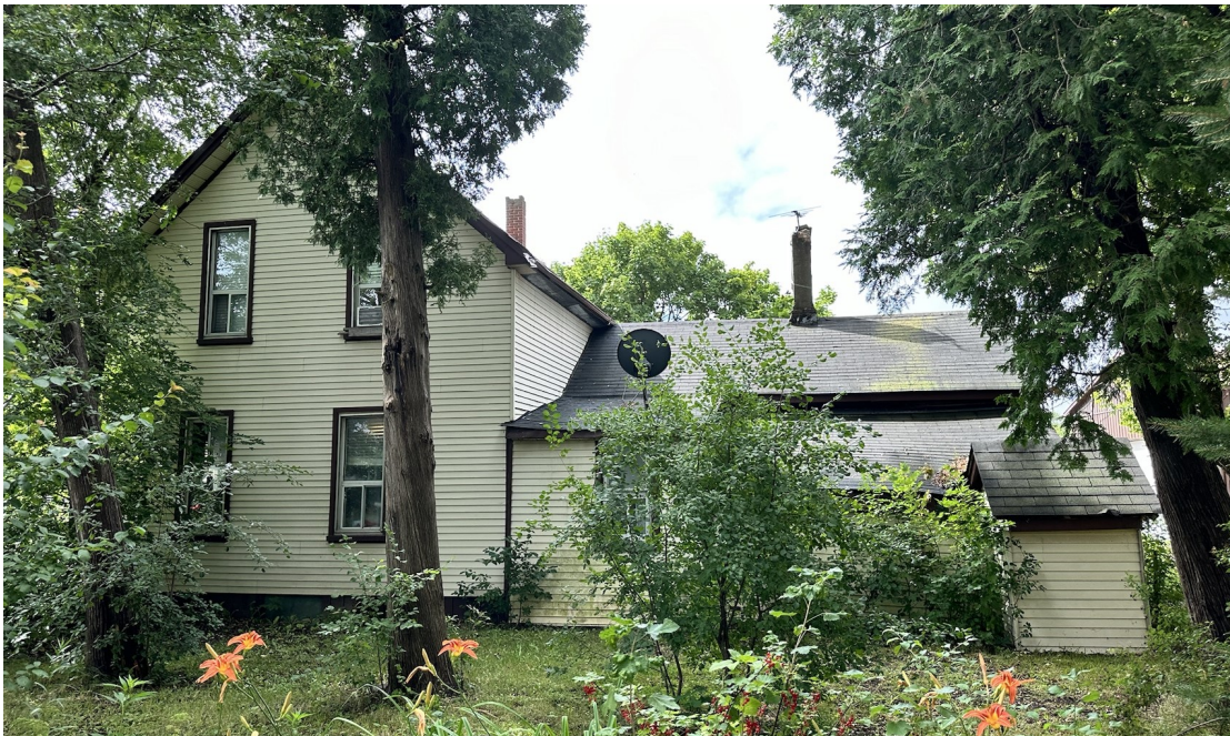
Figure 6 - Right Side (north) elevation of 11534 McCowan Road, Markham (LA)
