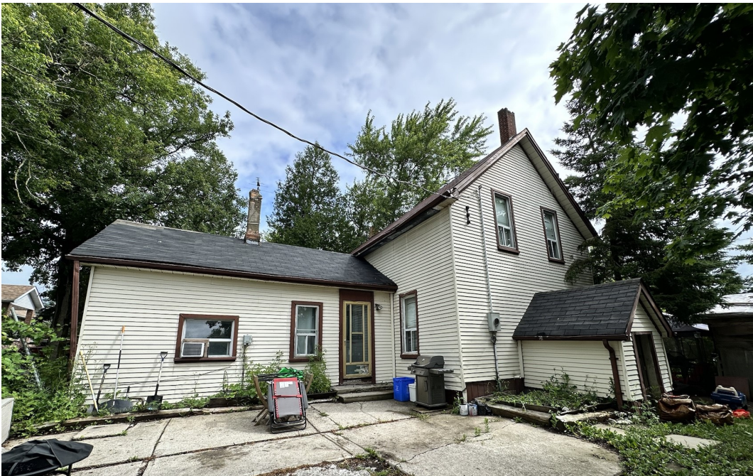
Figure 8 - Left Side (south) elevation of 11534 McCowan Road, Markham (LA)
