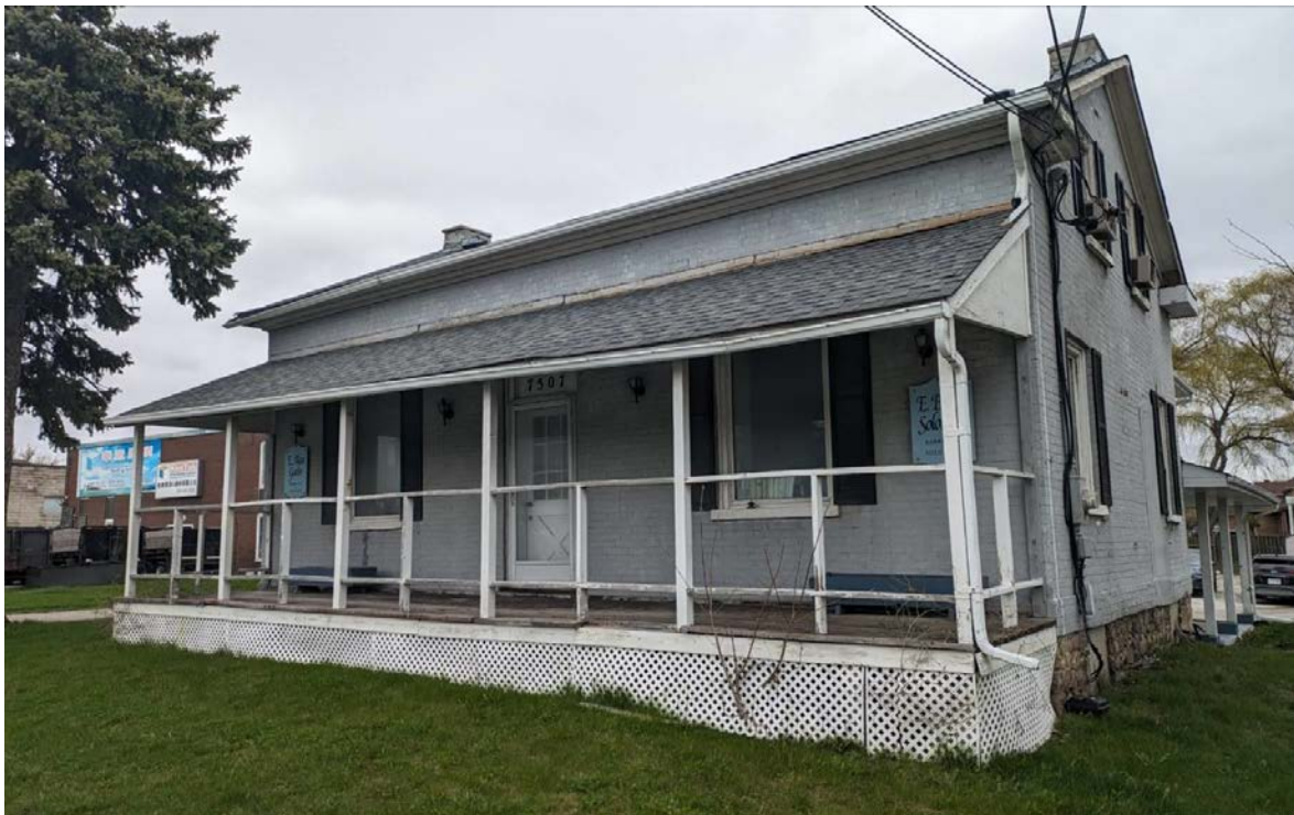
Figure 3 - Front (west) elevation of 7507 Kennedy Road, Markham
