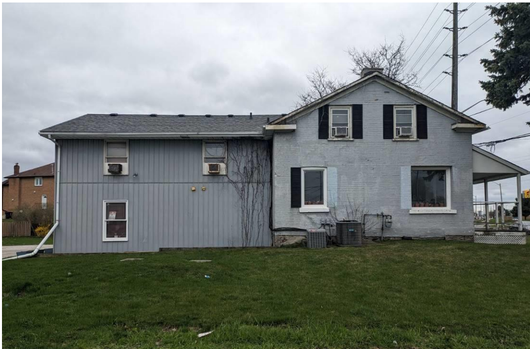
Figure 5 - North Elevation of the rear addition and original 1½ storey building.
