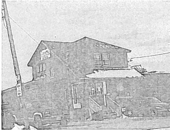
MacDonnell-Prentice House 58 Old Kennedy Road c.1925
