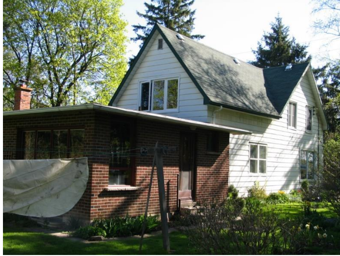
7696 Ninth Line. West and south side view showing rear wing and 1960s addition.
