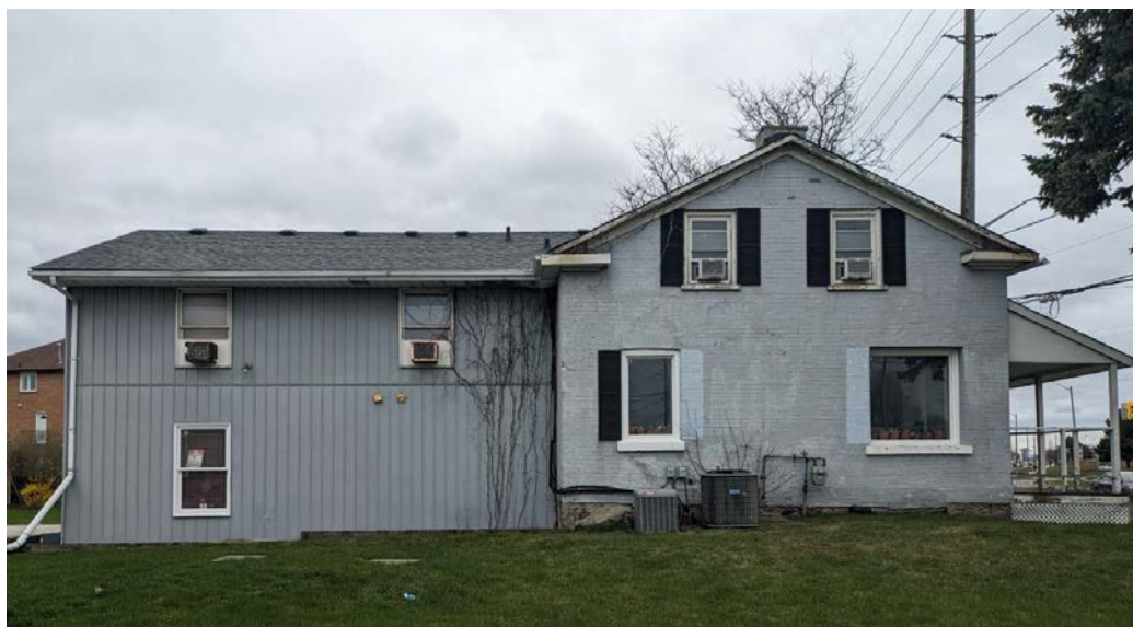
Figure 9 - The (left) side elevation of 7507 Kennedy Road (LA)
