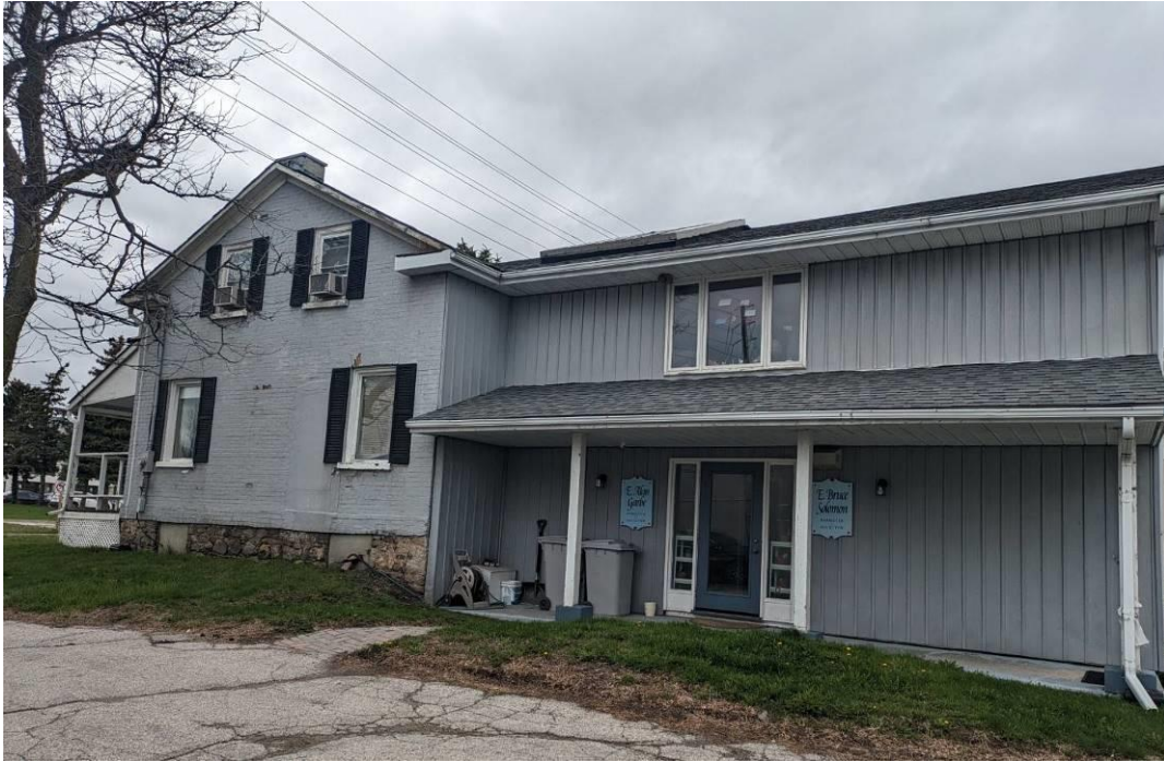
Figure 4 - South elevation of the original 1½ storey building and rear addition.
