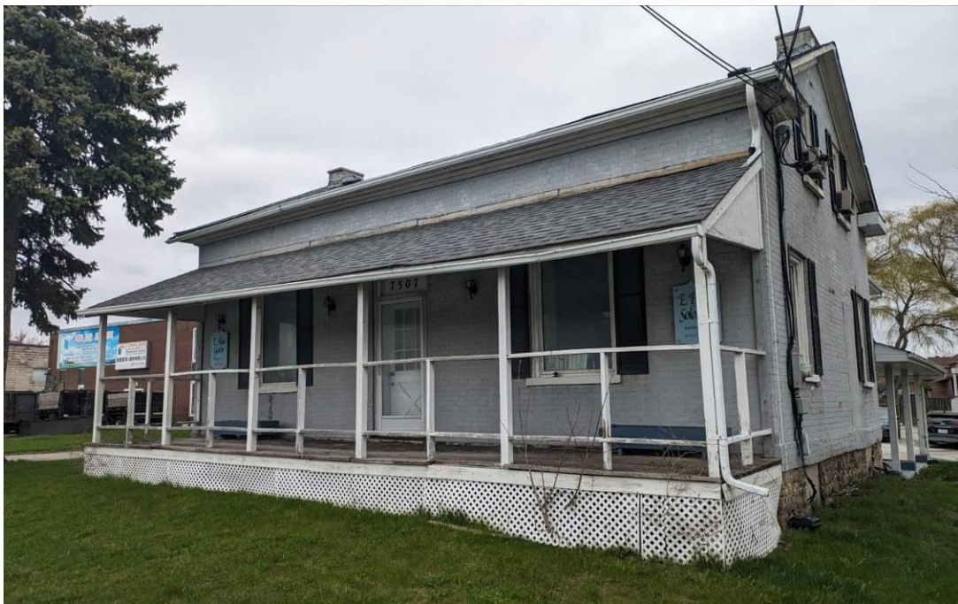
Figure 3 - Front (west) elevation of 7507 Kennedy Road, Markham
