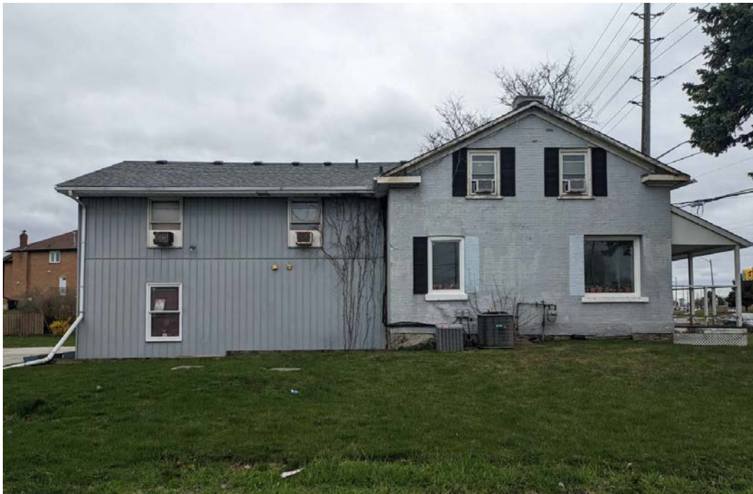
Figure 6 - North Elevation of the rear addition and original 1½ storey building.
