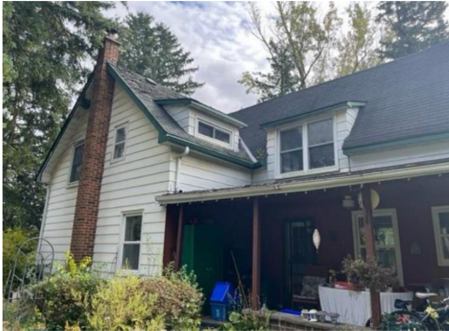
Figure 10 - The (right) side elevation of 7696 Ninth Line (Heritage Markham Memo Feb 2024)
