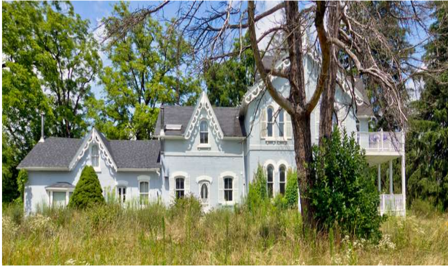
Heritage Dwelling and Addition - South Facade
