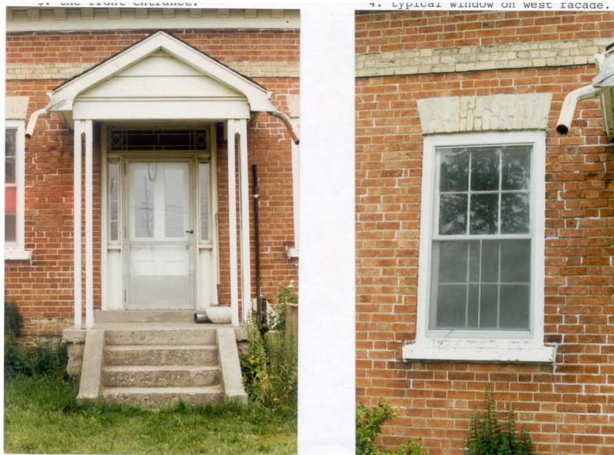
Front doorcase and typical window prior to alterations in 1990. Note geometrical glazing pattern of transom light.
