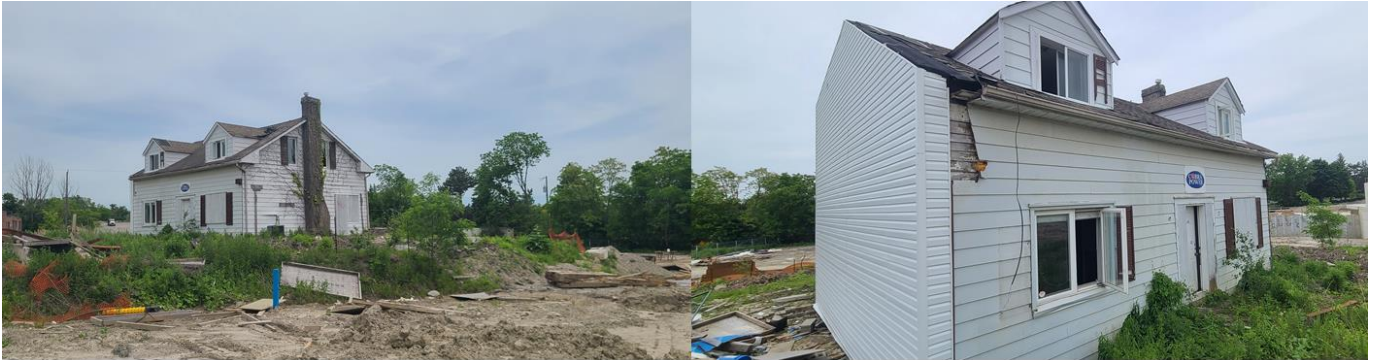
After the removal of the newer addition
