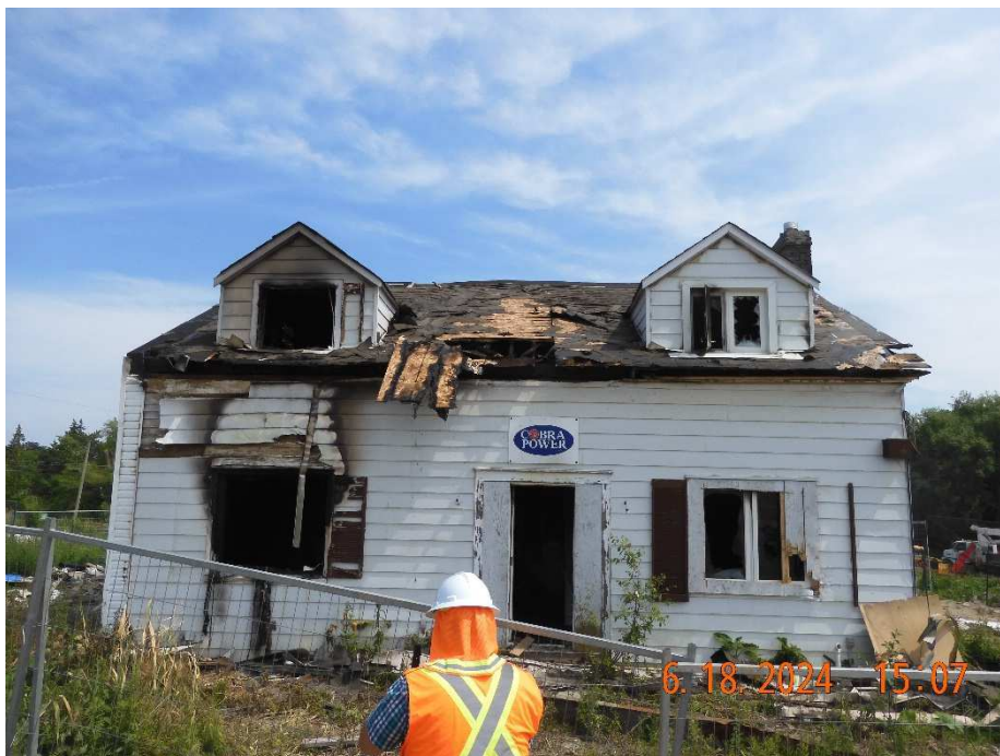
Roof deck @ south side of building
