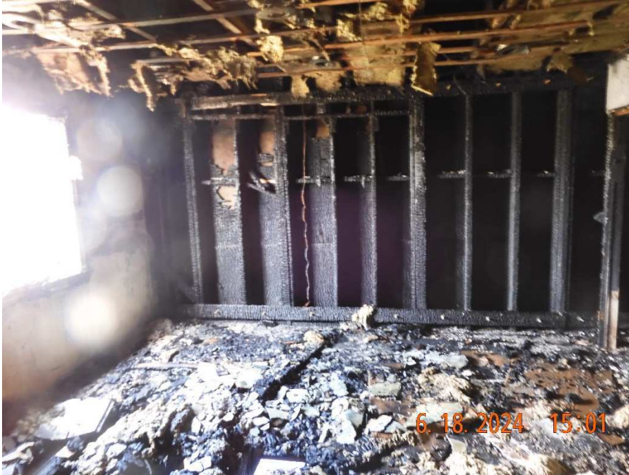
Wood stud wall frame @ east side (from inside & ground floor level)
