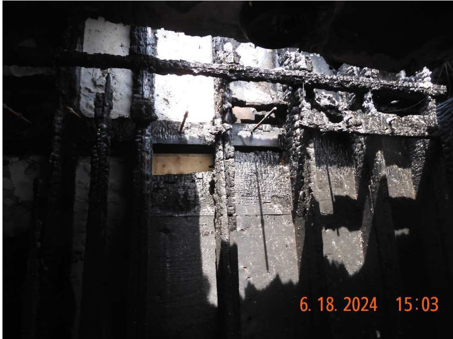
Wood stud wall frame @ east side (from inside & 2nd floor level)
