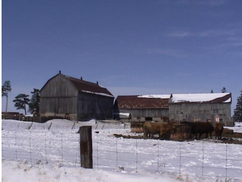
Barn complex at 9318 Reesor Road/7484 Sixteenth Avenue.
