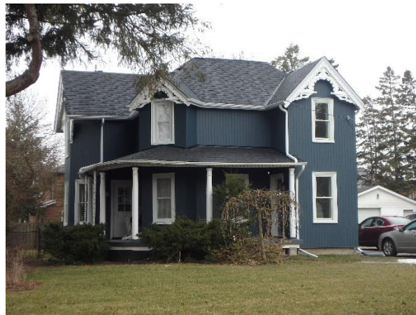
The Fretz House, 1904 at 36 Peter Street shares some design similarities with the Reverend Peter Cober House.
