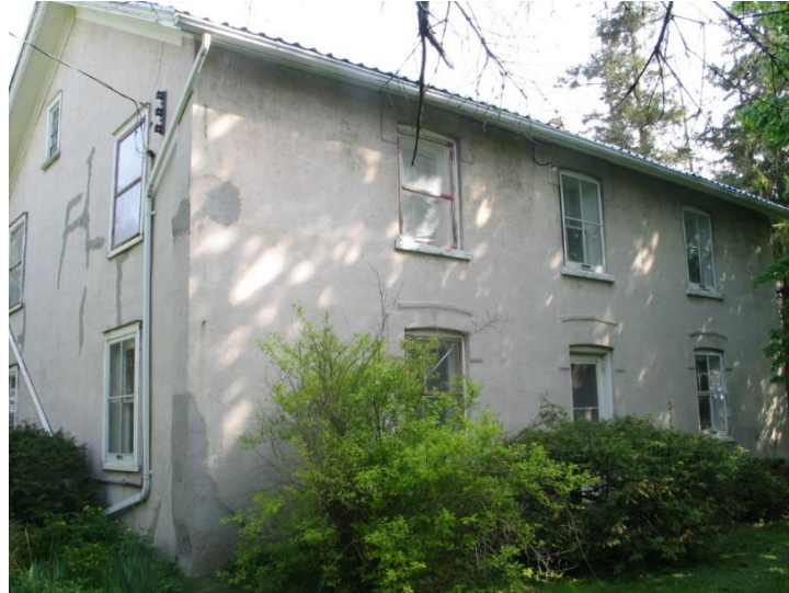
South and west views of 9318 Reesor Road. Note that the windows on the west gable end lack the Italianate “eyebrow” arches.
