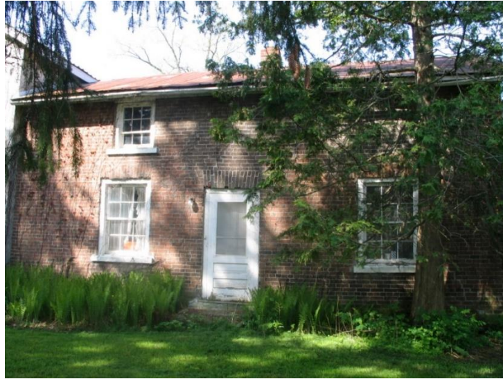
Brick wing of 9318 Reesor Road, an addition of the mid-1850s
