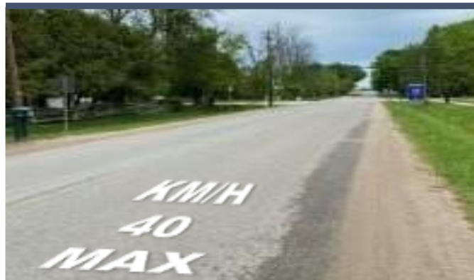
On-Road Pavement Markings
