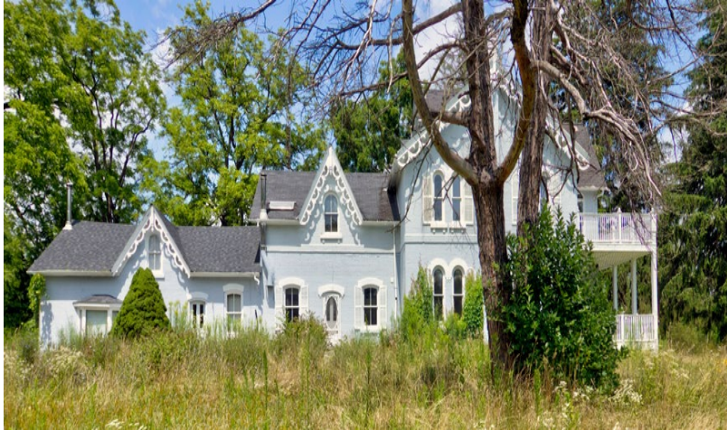
Heritage Dwelling and Addition - South Facade
