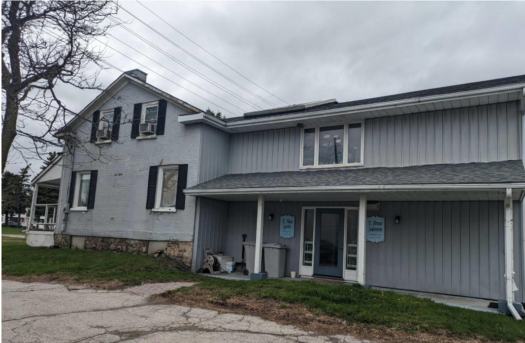
Figure 5 - South elevation of the original 1½ storey building and rear addition.
