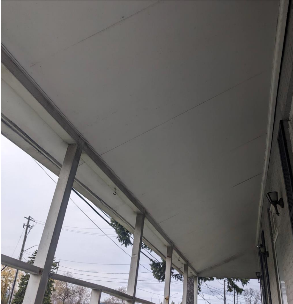
Figure 4 - View of Plywood Soffit below front veranda roof.
