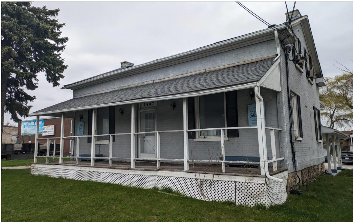
Figure 3 - Front (west) elevation of 7507 Kennedy Road, Markham
