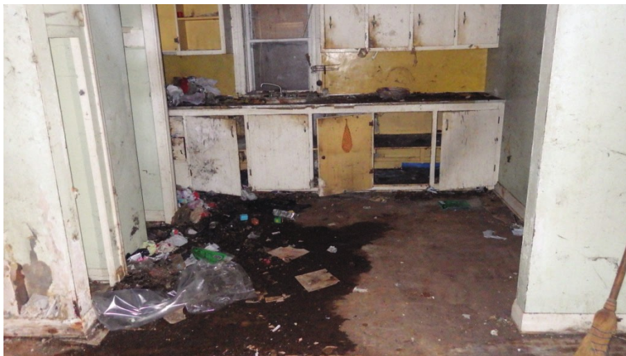
Figure 4 – The inside floor
