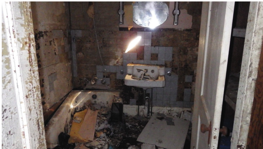
Figure 7 – Bath room area
