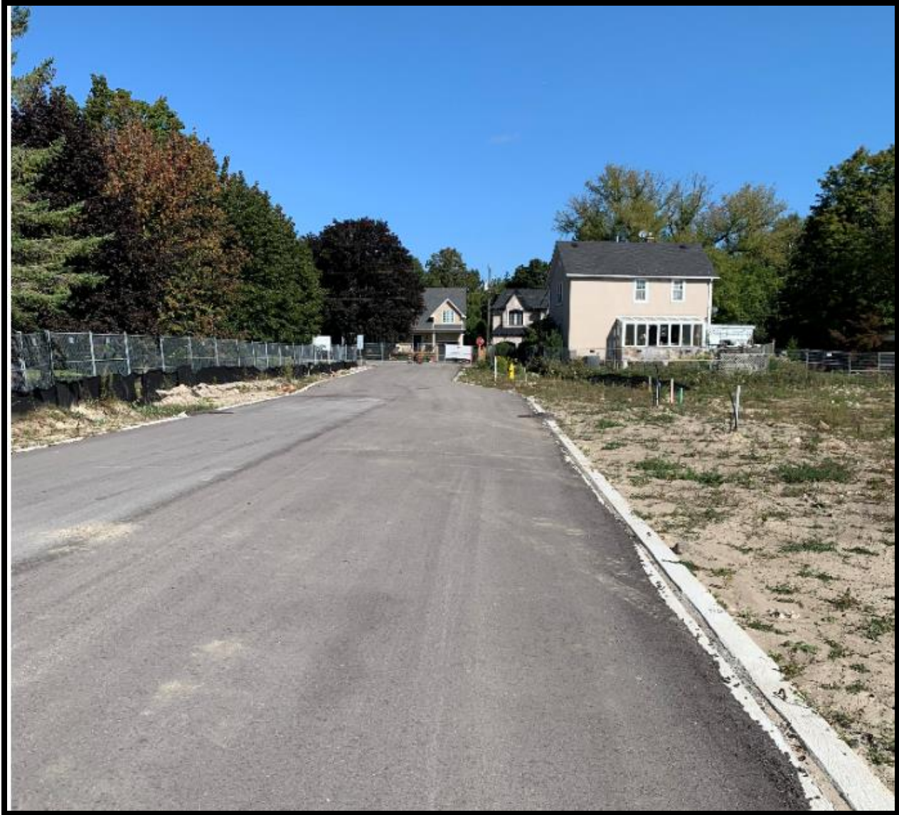
View of subject property looking north towards Parkway Avenue
