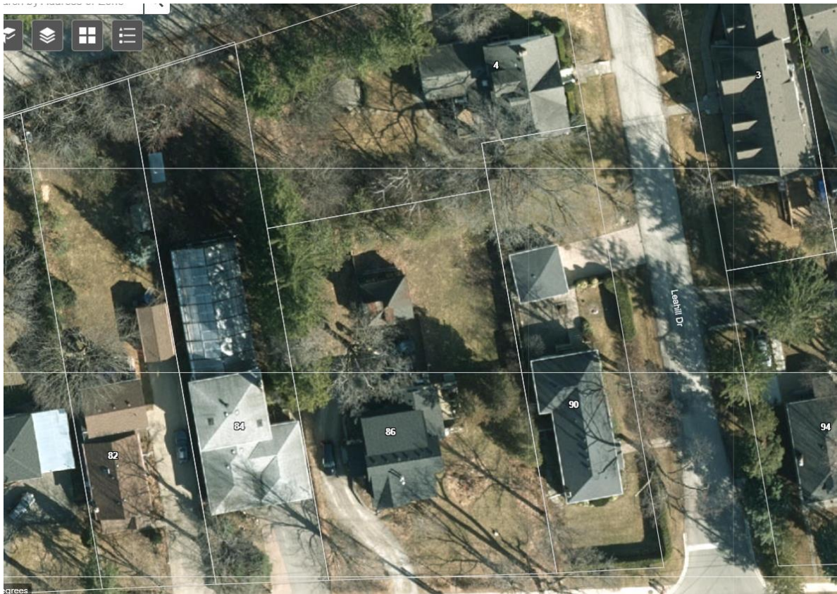
Figure 5 - An aerial view of the subject property and its neighbours. The houses adjoining 86 John Street are all 1 1/2 storey or less.
