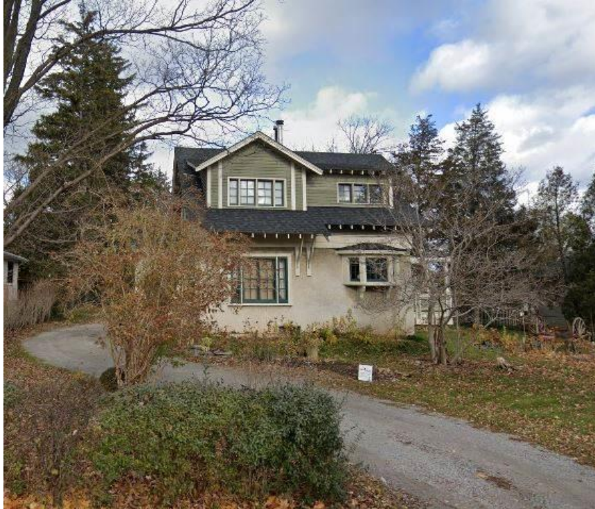
The south (primary) elevation of heritage dwelling on the Subject Property (Source: Google)
