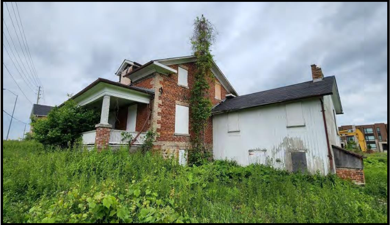
Historic one storey east addition built into existing slope
