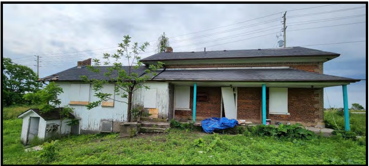
Historic Rear Veranda
