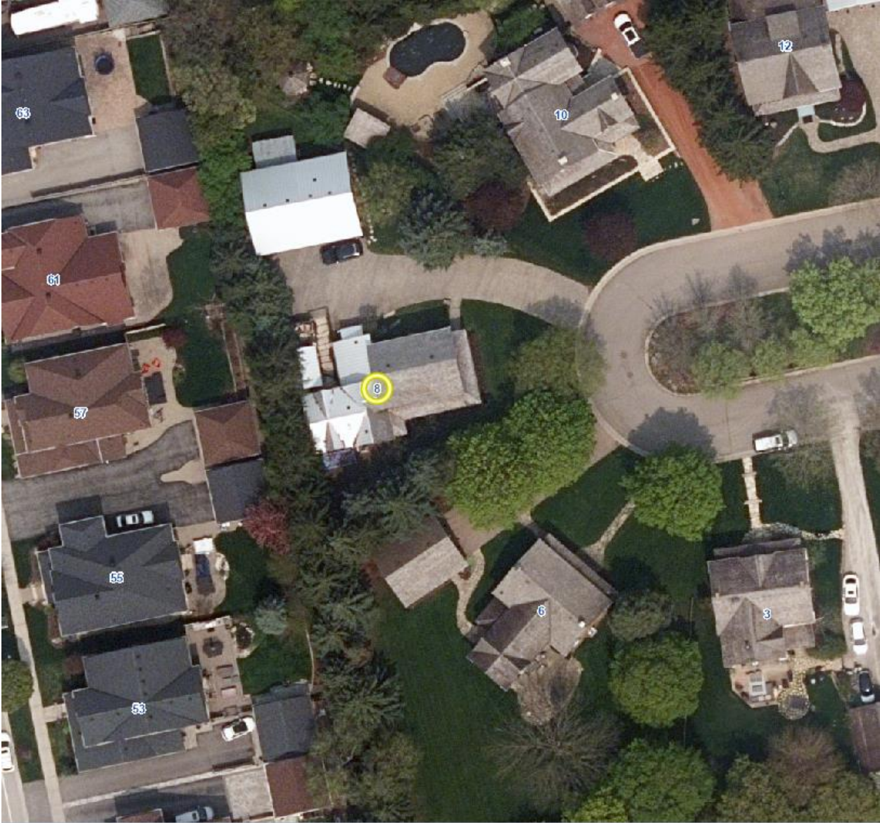
Aerial View of metal roof installed at 8 David Gohn Circle
