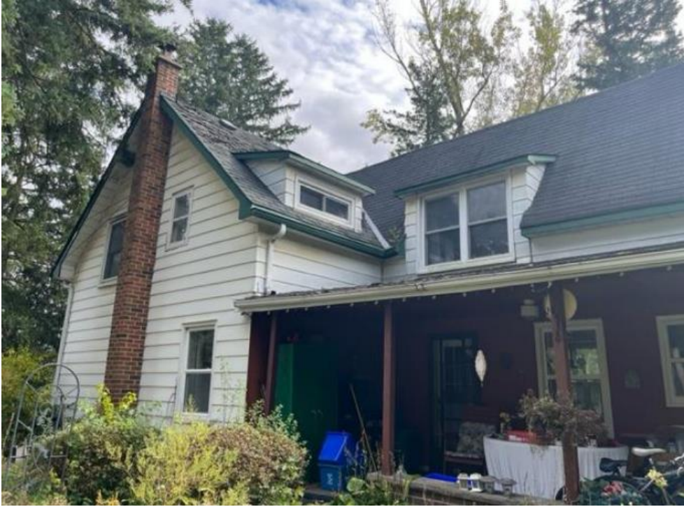
The north elevation of the on-site dwelling as seen in October 2023 (Source: Applicant)
