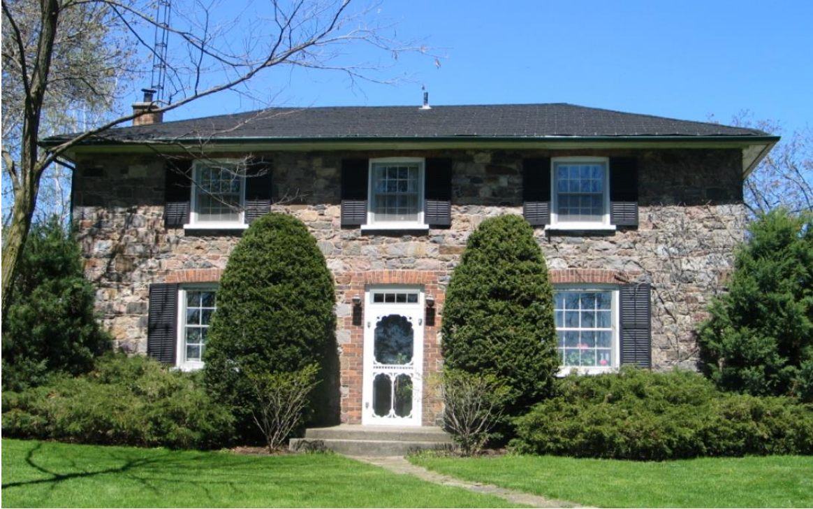
Attachment B- Photograph of Graham-Hallman House Prior to installation of metal roof 2004
