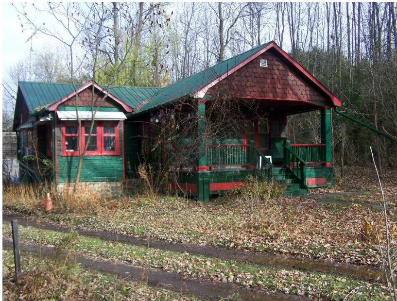
6084 Nineteenth Avenue in 2013, before renovations and addition to rear.
