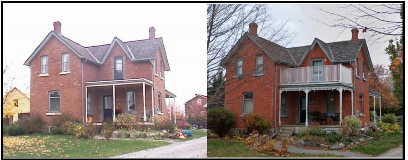
The same house before and after a wooden code compliant railing added to roof of veranda
