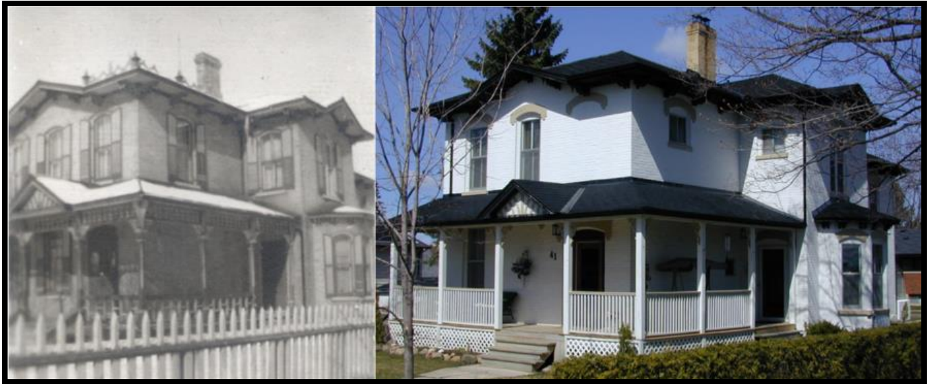
Archival and contemporary photo of the same house with original historic railings and code compliant wooden railing.
