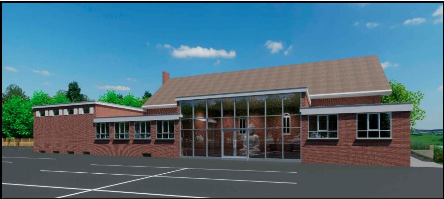
View looking South
