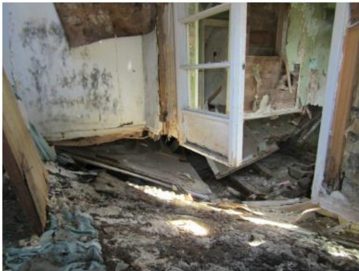
Photo No. 4: Collapsed ground-floor structure
