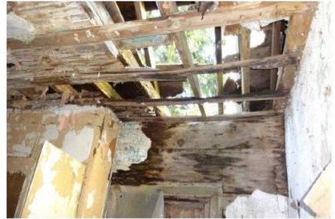
Photo No. 3: Addition - Hole in Roof
