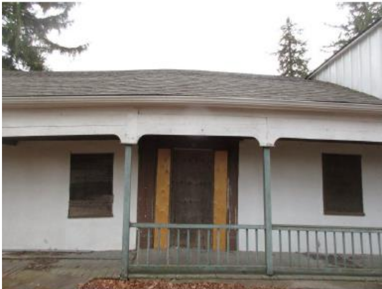
Photo No. 2: North elevation - leaning to the west
