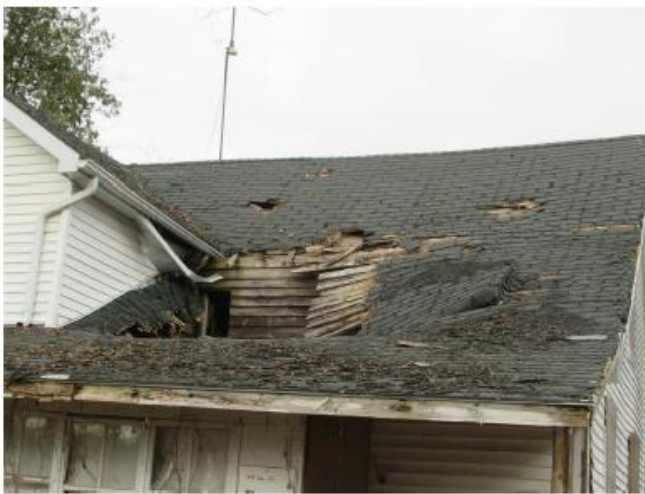
Photo No. 5: Collapsed roof structure from exterior
