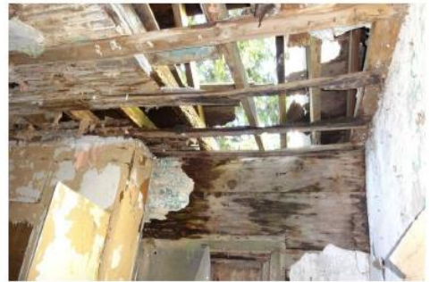
Photo No. 3: Addition - Hole in Roof
