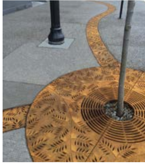
Buchart Horn Architects and Engineering. Locust 6' Dia. tree grate installed with 12" trench arrayed on various radii. Etna, PA.
