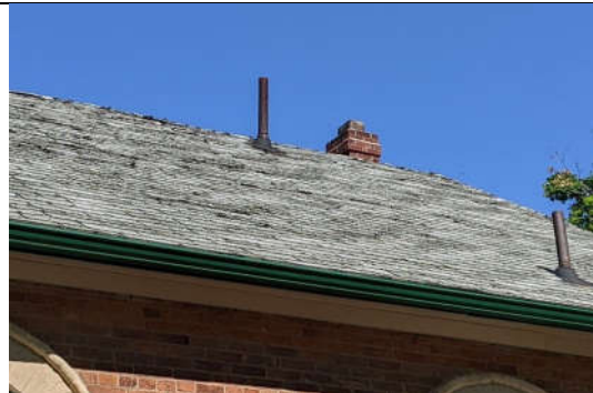
Photo 2: Degranulation and curling of shingles at roof.
