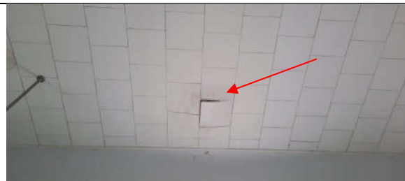
Photo 5: Leaking at building interior, significant leak event to cause this "bubbling" of the tile.
