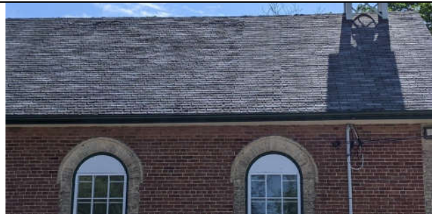
Photo 2: Degranulation and curling of shingles at roof.
