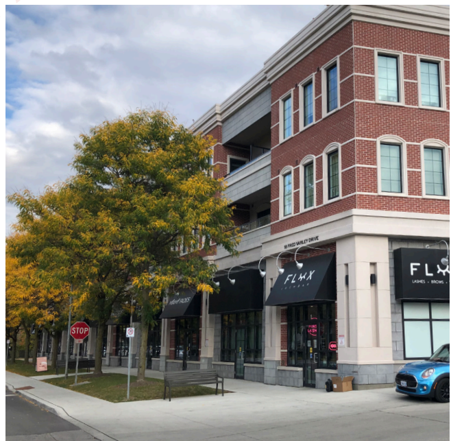
Figure 87. This mixed use development in Unionville is setback further from the street to afford an expanded sidewalk for additional landscaping and seating.
