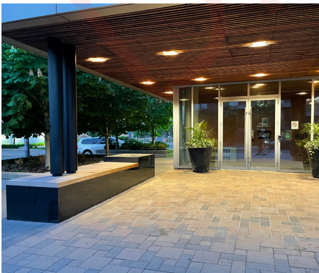
Figure 67. This building entrance is well-lit, weather protected and provides higher bench seating heights suitable for older adults.
