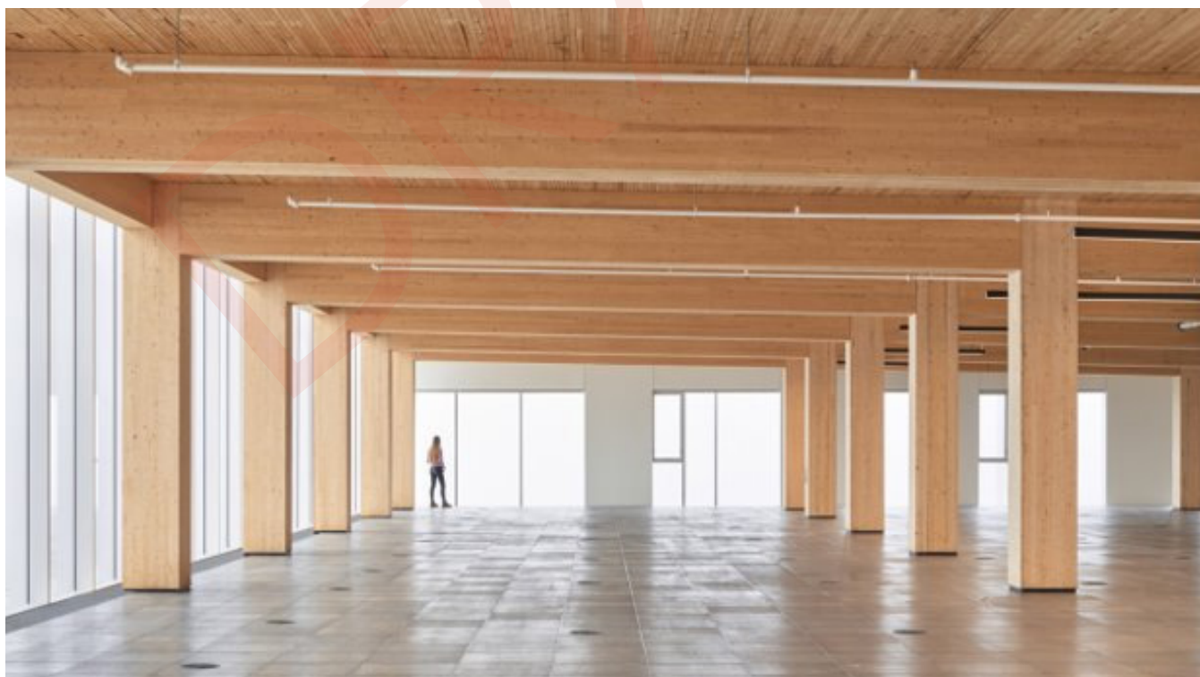
Figure 61. Wood-frame construction affords added flexibility when designing low or mid-rise apartment buildings.
