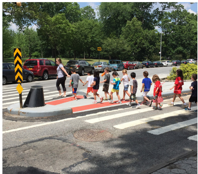
Figure 25. This refuge island in New York helps to shorten the crossing distance while providing a place to rest.
