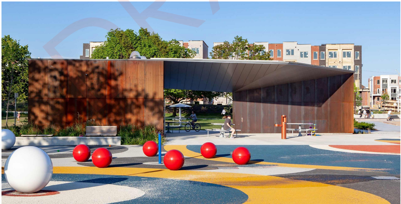
Figure 48. These washrooms in Stanley Greene Park in North York also provide a water station and weather protected seating.
