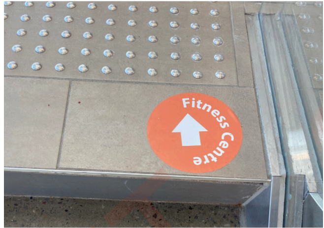
Figure 75. Tactile features at the top of a common stairway with integrated wayfinding.
