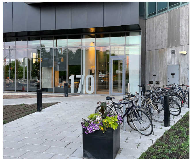
Figure 68. This development provides bicycle parking with clear sight lines to the seating area in the lobby for natural surveillance.
