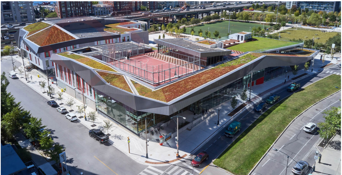
Figure 5. Canoe Landing Campus in Toronto co-located two elementary schools, a community centre, child care, and a publicly accessible open space adjacent to a public park.
