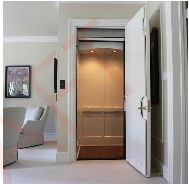
Figure 116. This elevator was retrofitted in an existing unit by making use of two closets stacked on top of each other on both levels.
