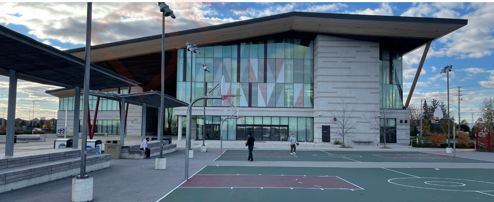
Figure 88. An animated edge with seating, weather protection, bicycle parking, and recreational facilities at Aaniin Community Centre.
