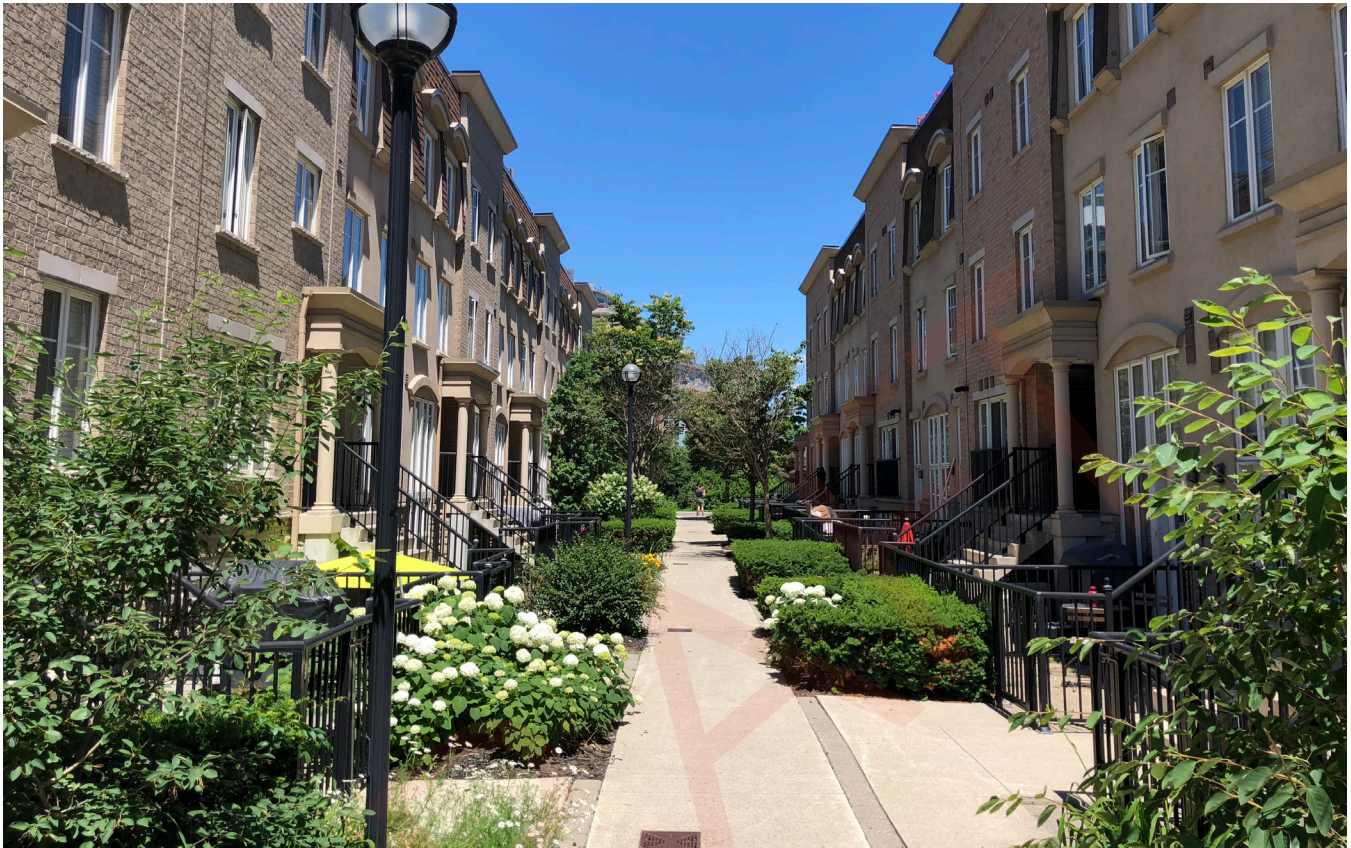
Figure 23. This pedestrian mews in Toronto provides access to townhouse units while providing a safe neighbourhood connection for pedestrians.
