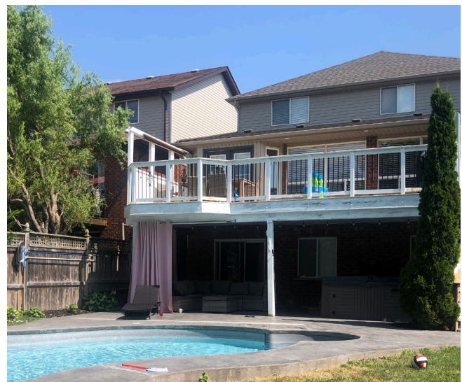
Figure 55. This house sited on a slope is afforded a no-step access to a basement level that has high ceilings and ample light.
