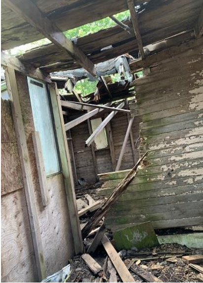
Rear tail of building- roof collapse (Heritage Section Photo)
