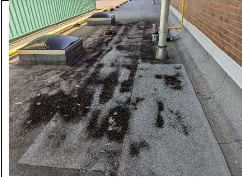
**Photo 1:** Numerous Blisters (elevated areas) in a high traffic area. Previous patch repairs (lighter coloured membrane areas).
