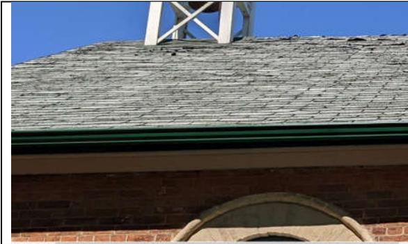
**Photo 1:** Roof shingles are curling at west elevation. Sign of UV degradation.
