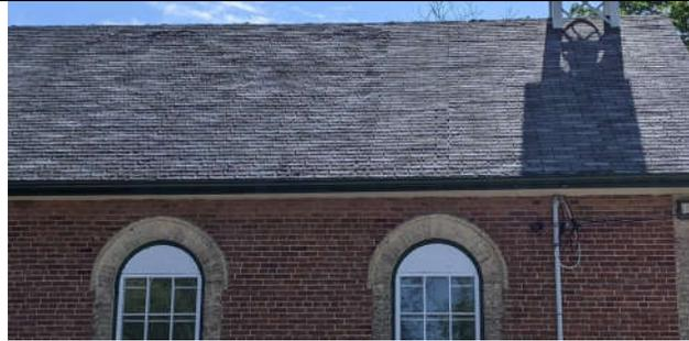
**Photo 4:** Shingle curling at the east elevation.
