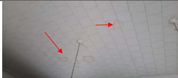
**Photo 6:** Water staining at the building interior.
