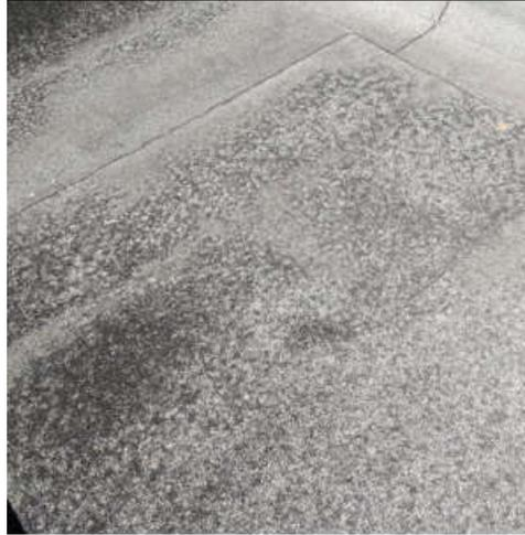
Photo 8: Roofing membrane degranulation. Granules protect roof from UV degradation.
