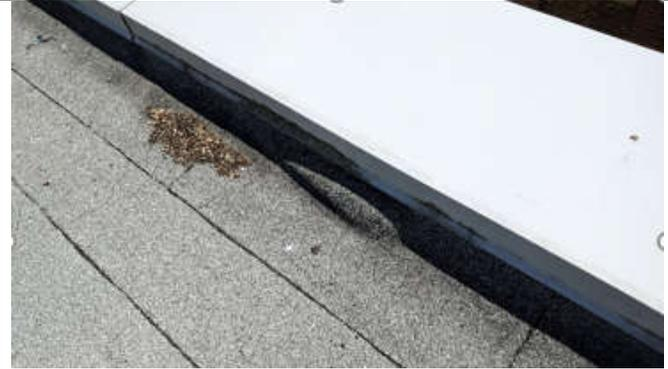
**Photo 4:** Blister at the roof perimeter. Note with increase in temperature blisters become larger this increases the thermal expansion/contraction of the membrane. This will increase wear on the membrane (e.g. degranulation, cracking).
