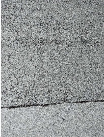
Photo 7: Alligatoring (cracking) of roofing membrane.
