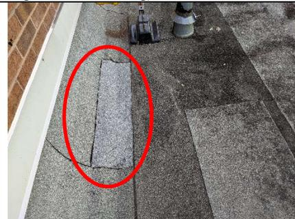
**Photo 6:** Previous patch repairs.
