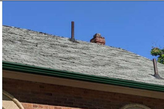
**Photo 2:** Degranulation and curling of shingles at roof.
