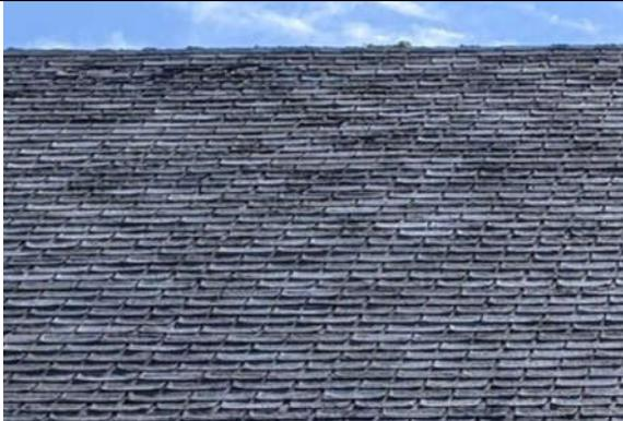
**Photo 3:** Widespread curling of the roofing shingles. Roof has failed.
