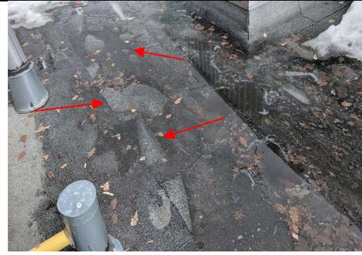
**Photo 2:** Close up of blister on Roofs at the same area as Photo 1. Significantly more blisters than what would be seen on a roof such as this.
