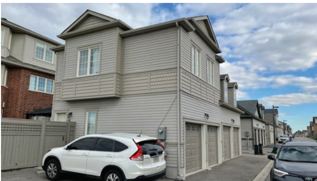
Figure 20. Laneway housing in Cornell
